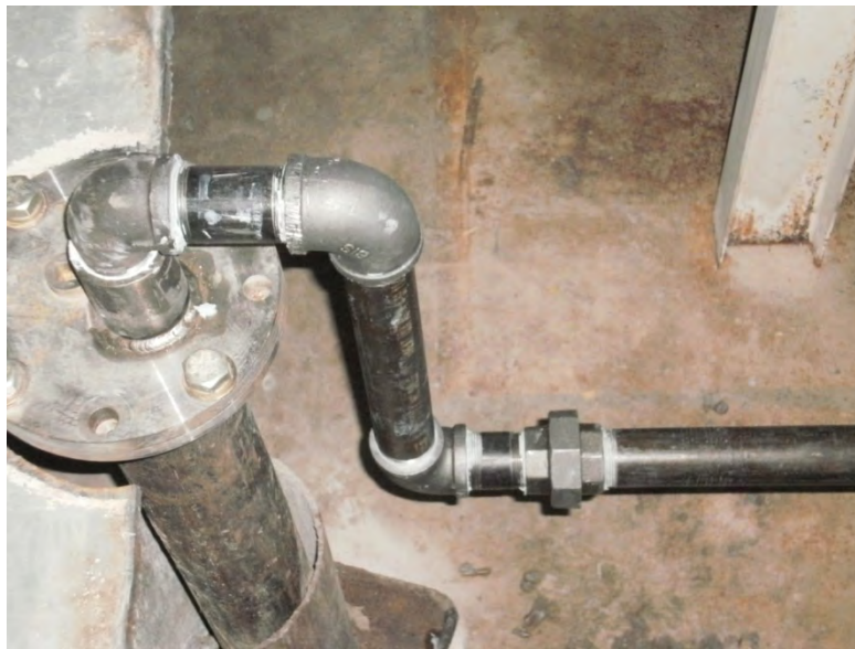
Photo 3.2 – Wellhead construction for AOC-SIW01.
