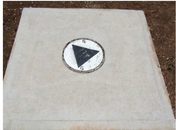
Photo 2.4 – Surface completion for CS-MW36-LGR.
