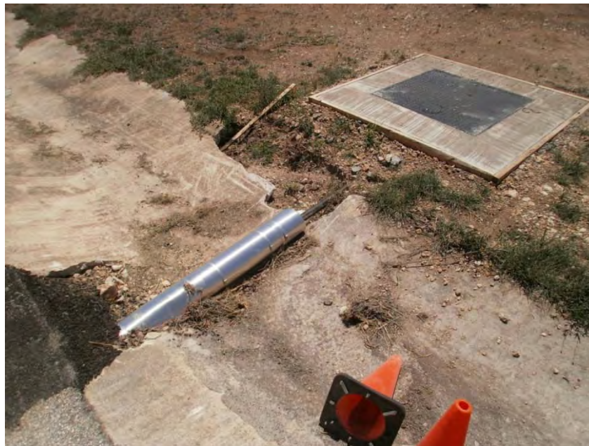
Photo 3.4 – Vault covering AOC-SIW01.
