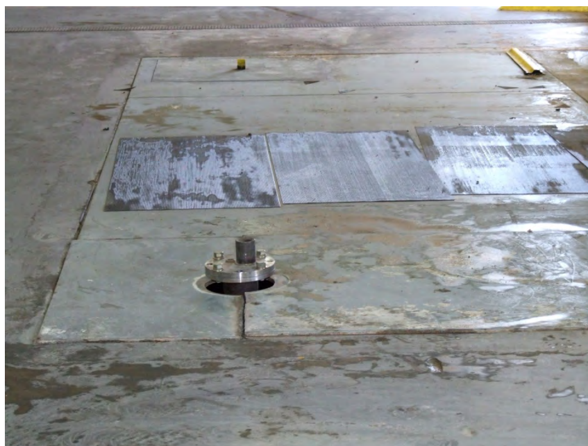
Photo 3.1 – Modified steel plate surrounding completed AOC-SIW01.
