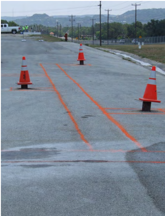
Photo 3.4 - AOC-65 asphalt prior to trenching.
