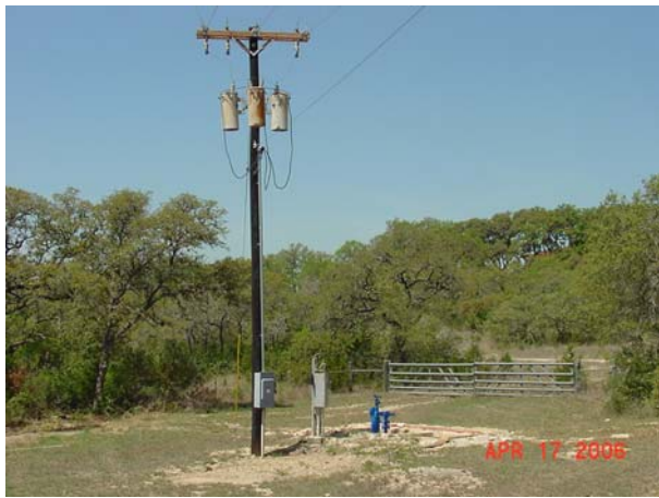
Well CS-9 before rehabilitation
