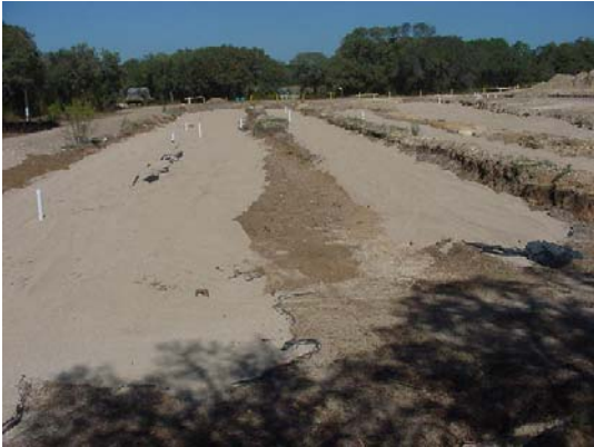
Bioreactor Trenches looking north
