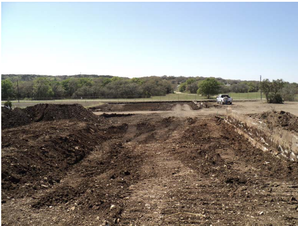
Photo 2. Excavation process, looking west.
