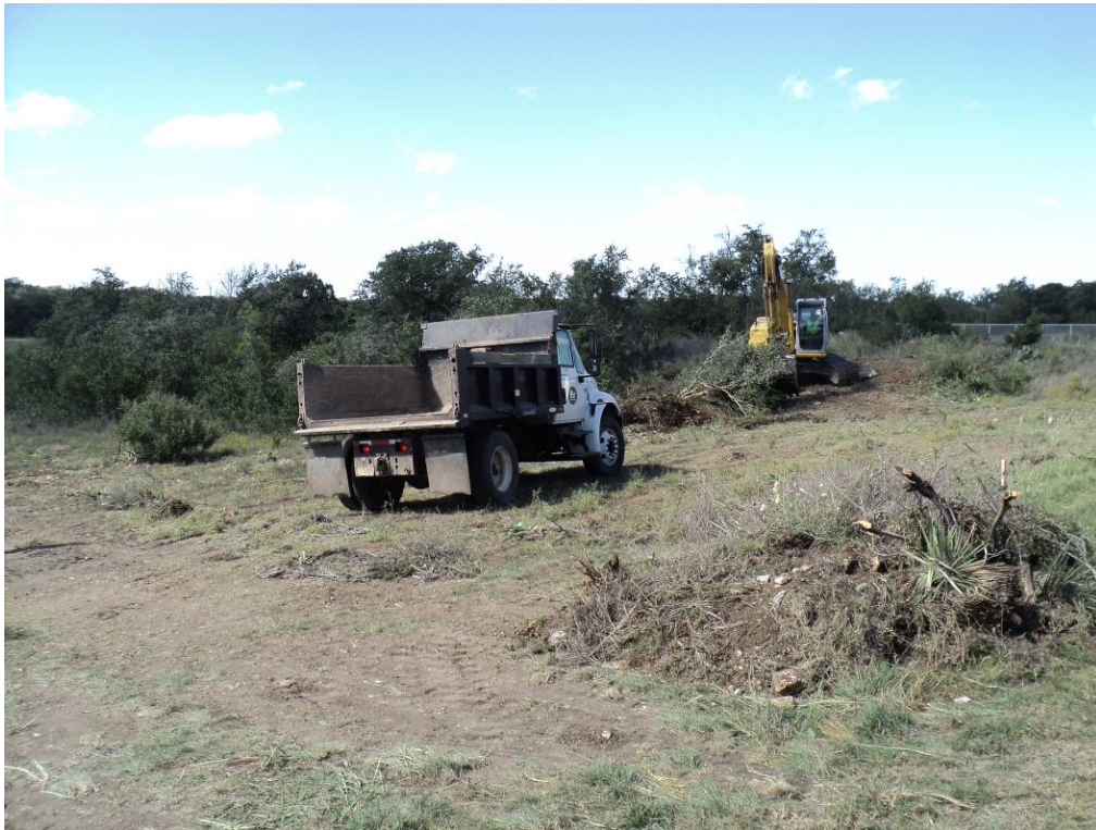
Photo 1. Clearing trees and brush.
