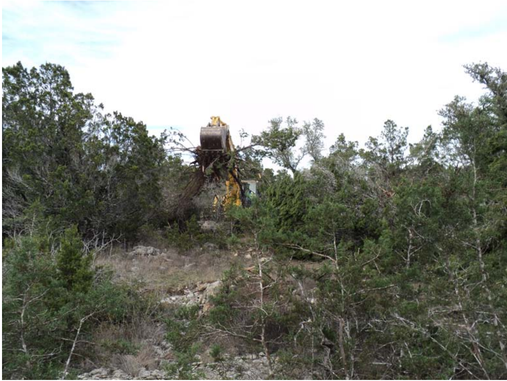
Photo 1. Pre-excavation vegetation removal.
