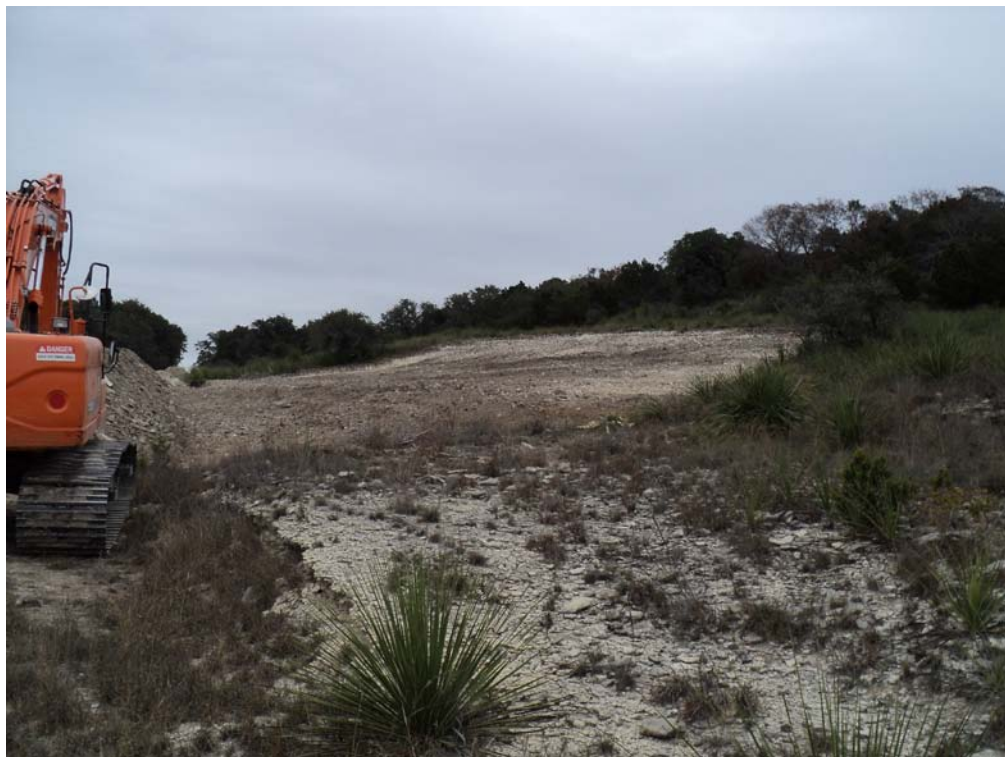
Photo 2. Top portion of excavation, looking north.
