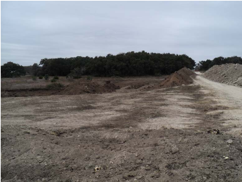
Photo 3. Bottom portion of excavation, looking north.
