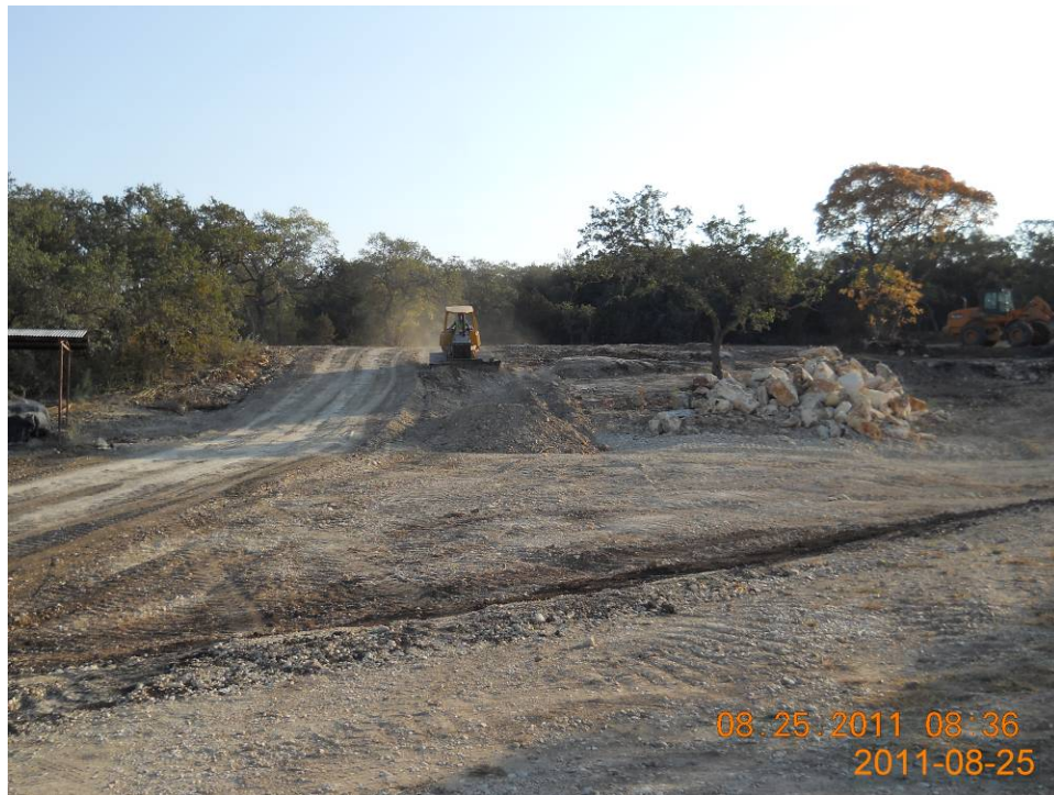
Photo 7. SS19 area at RMU-2 after overexcavation, looking north (August 2011).
