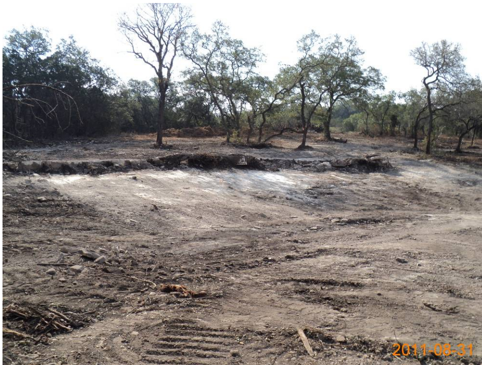
Photo 8. SS67 area at RMU-2 after overexcavation, looking east (August 2011).
