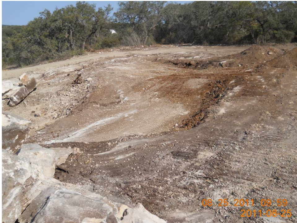
Photo 9. SS65 and SS70 area at RMU-2 after overexcavation, looking west (August 2011).
