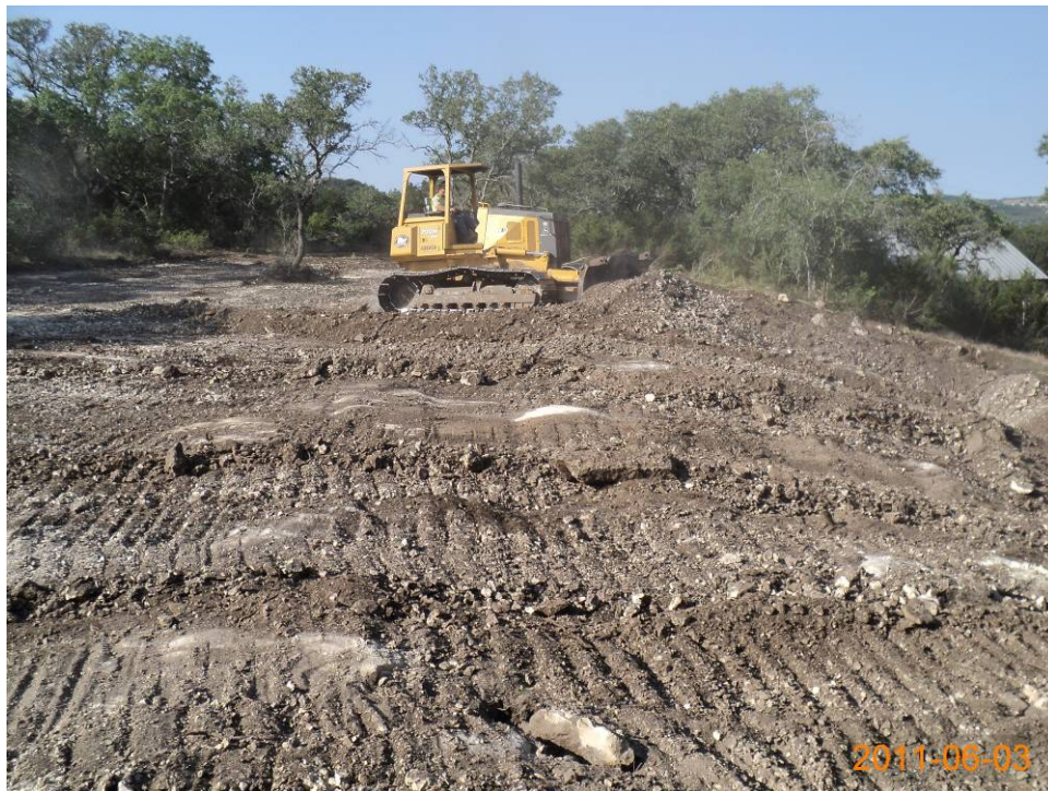
Photo 5. Excavation on top of berm at RMU-2, looking south (June 2011).
