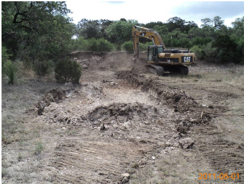
Photo 3. Initial excavation at RMU-2, looking east (June 2011).
