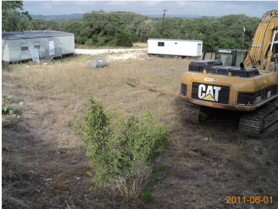
Photo 1. RMU-2 prior to excavation, looking west (June 2011).
