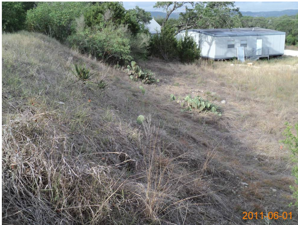
Photo 2. RMU-2 berm prior to excavation, looking south (June 2011).
