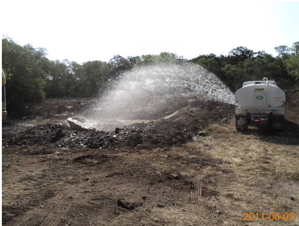
Photo 11. Adding water to excavated soil for dust control, looking east (June 2011).
