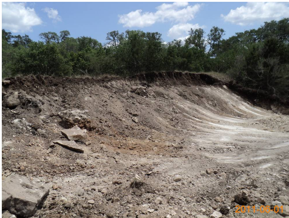
Photo 6. RMU-2 Berm after excavation, looking east (June 2011).
