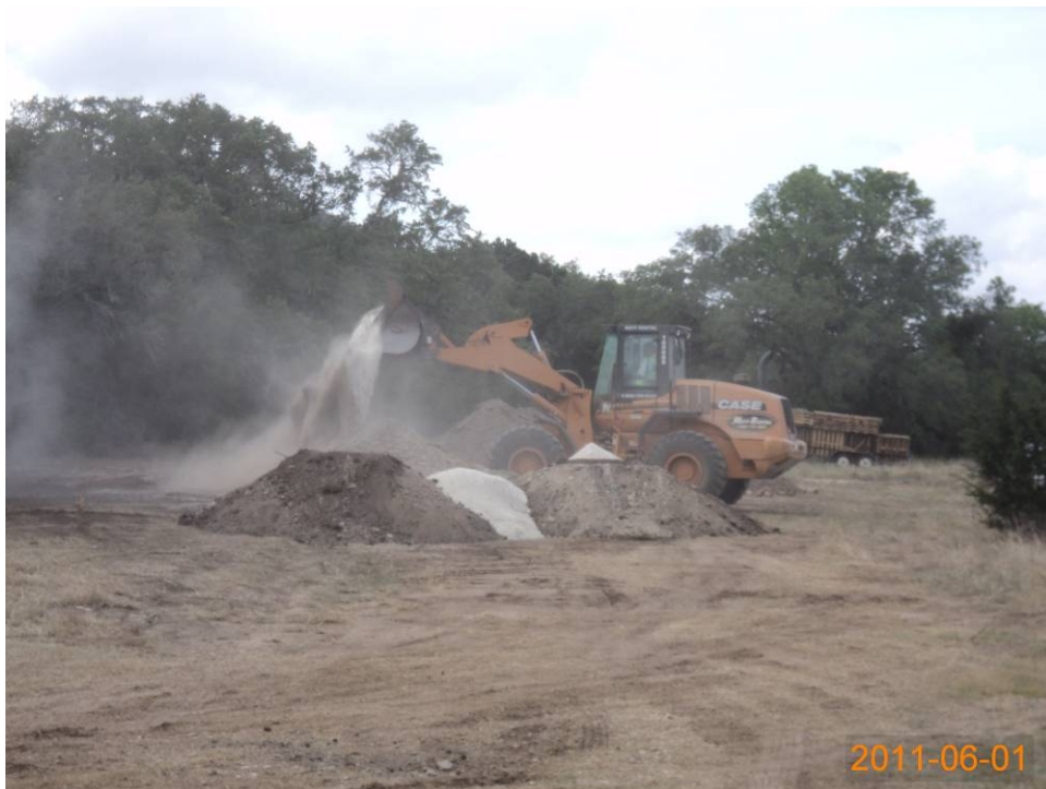
Photo 10. Mixing PIMS with excavated soil at RMU-2, looking west (June 2011).
