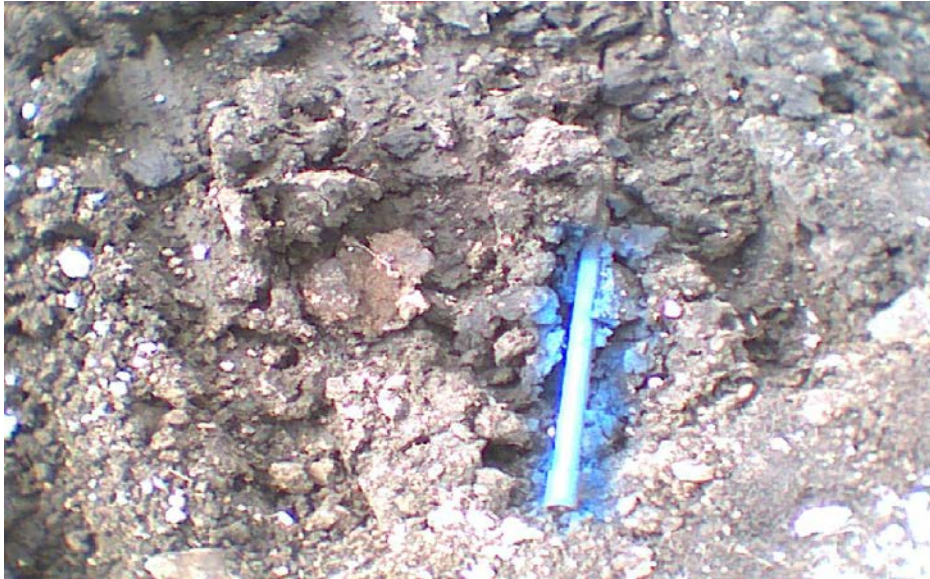
Anomaly ID LR-100 (Old utility line)
