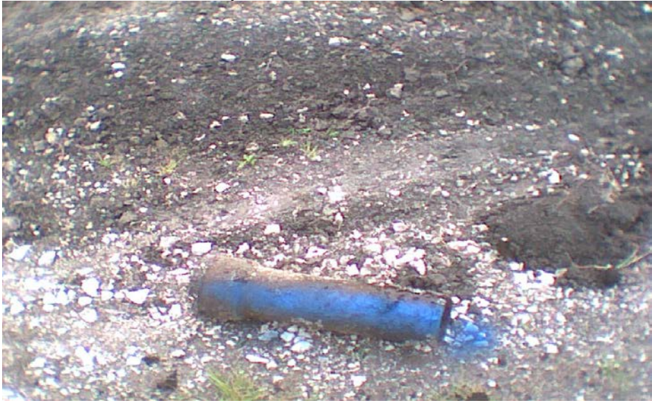
Anomaly ID LR-066 (Old utility line)
