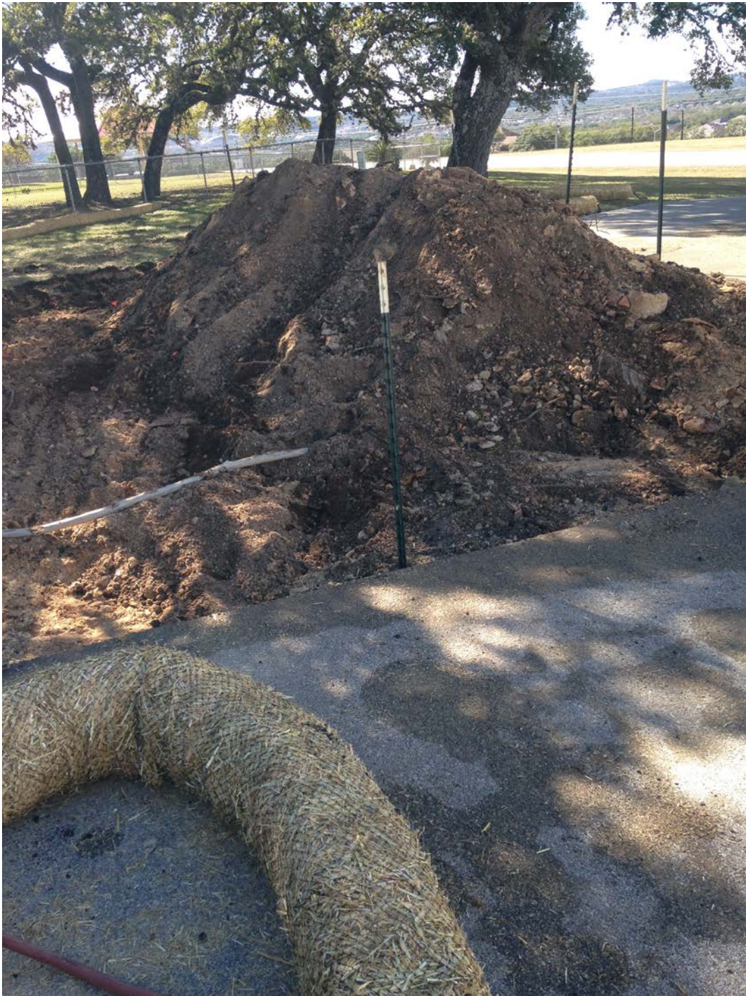
Photo 1. Excavation of soil material at AOC-76, looking east.
