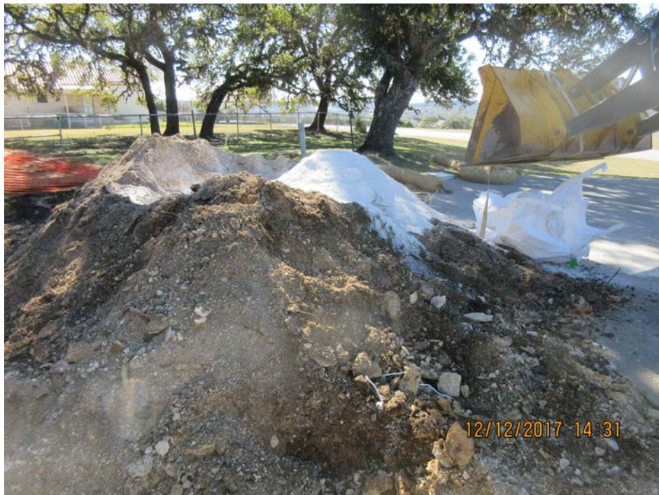
Photo 3. Treating excavated soil for reuse at East Pasture Berm.
