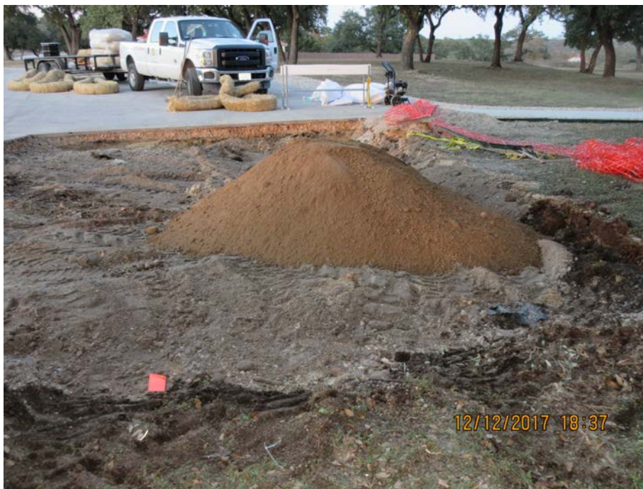
Photo 5. Backfilling excavation with clean soil.
