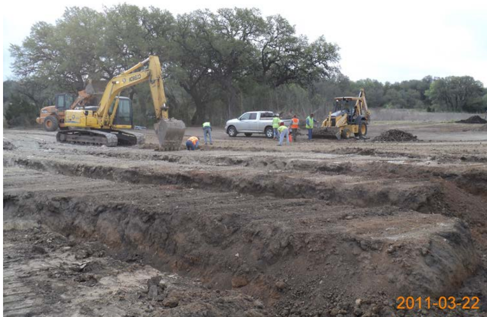
Photo 11. Excavation of AOC-62, looking northwest (March 2011).
