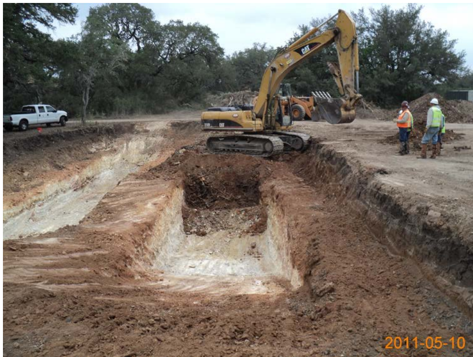
Photo 6. Excavation of Trench 2 at AOC-52, looking north (May 2011).
