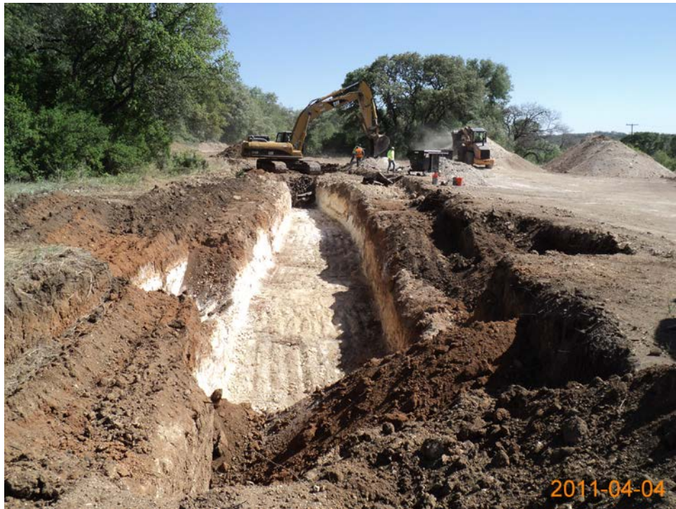
Photo 1. Excavation of Trench 1 at AOC-42, looking south (April 2011).
