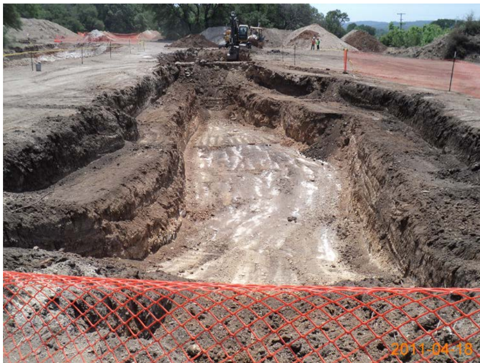
Photo 2. Excavation of Trench 2 at AOC-42, looking south (April 2011).
