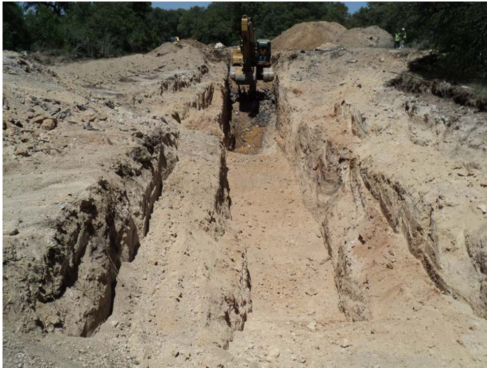
Photo 9. Excavation of AOC-58, looking south (May 2011).
