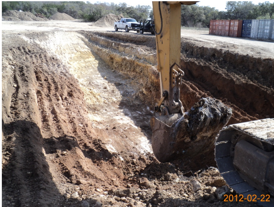
Photo 1. Excavation of the new trench at SWMU B-4, looking south (February 2012).
