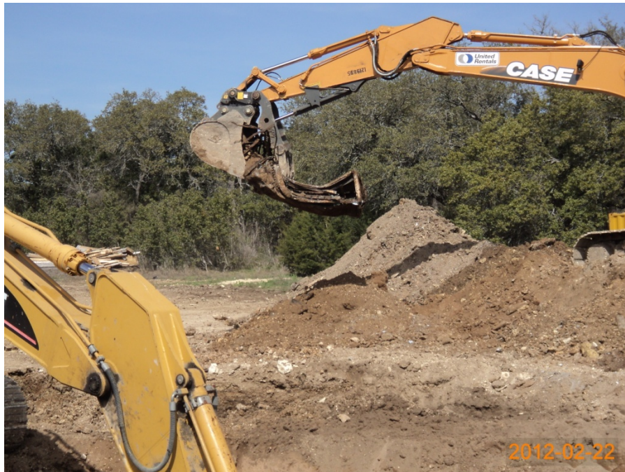
Photo 3. Excavator sorting metal debris at SWMU B-4, looking east (February 2012).
