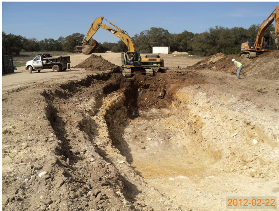
Photo 2. Excavation of the new trench at SWMU B-4, looking north (February 2012).
