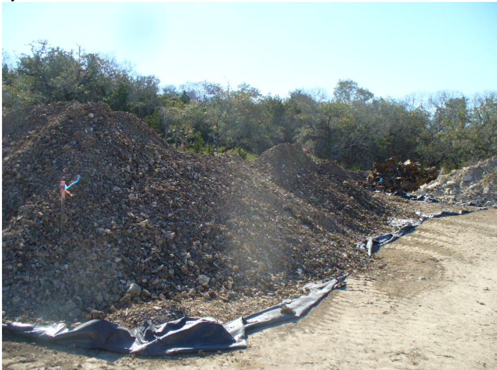
19. Separated debris and rock. View to southeast, February 2011.
