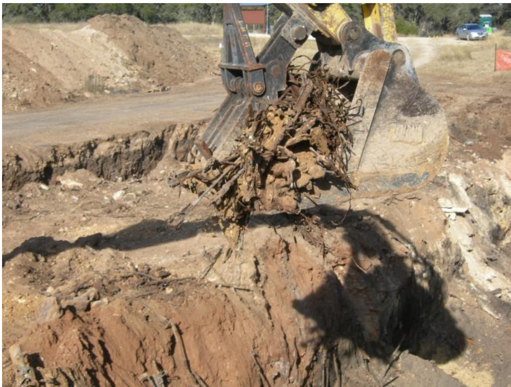
6. Debris (e.g., small arms barrels, metal banding), Trench Ca. View to north, January 2011.
