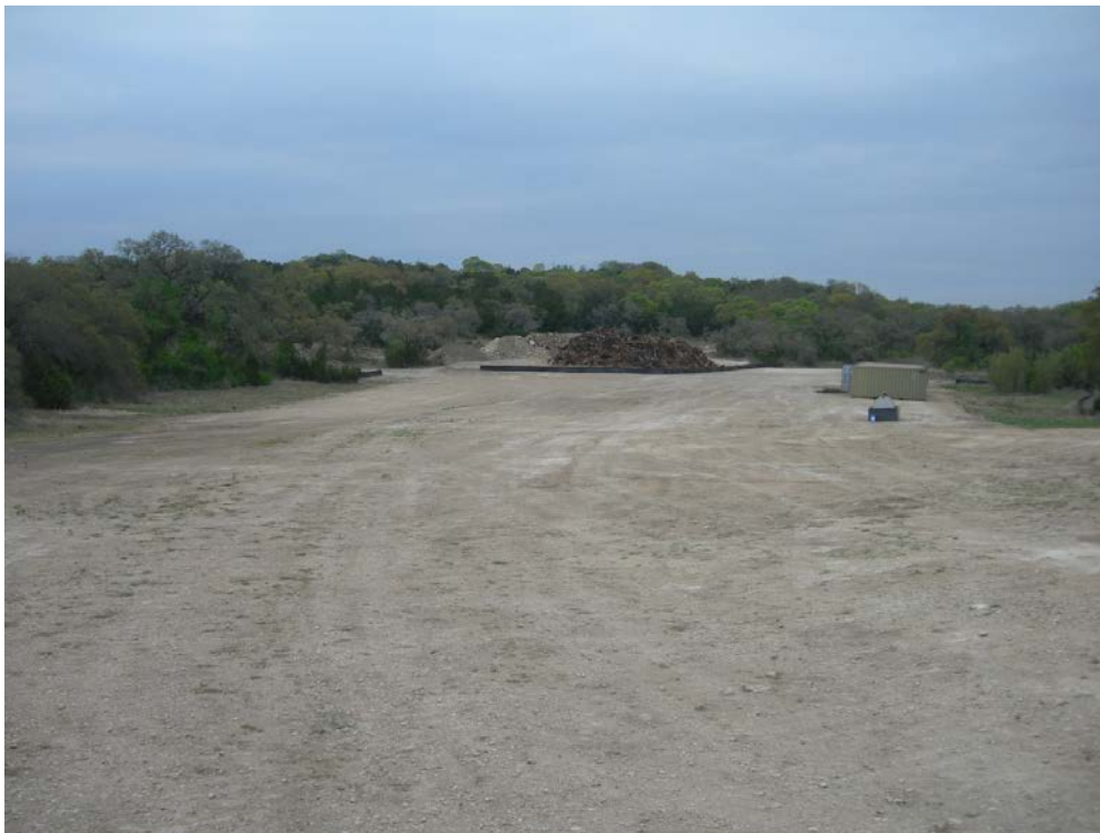
21. SWMU B-4 after surface scraping and grading. Stockpile area behind silt fence in background. View to south, March 2011.
