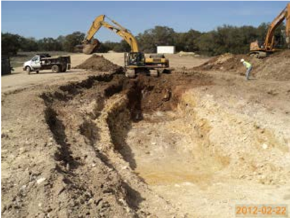
24. Excavation of Trench NT1. View to north, February 2012.
