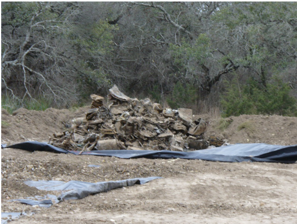
17. Large metal segregated for potential recycling. Stockpile area, southeast SWMU B-4. Earthen stormwater berm visible in background. February, 2011.
