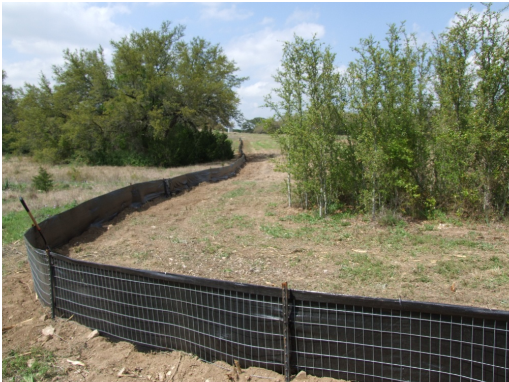
2. Silt fence installed along down-slope southern and eastern site perimeter, April 2010.
