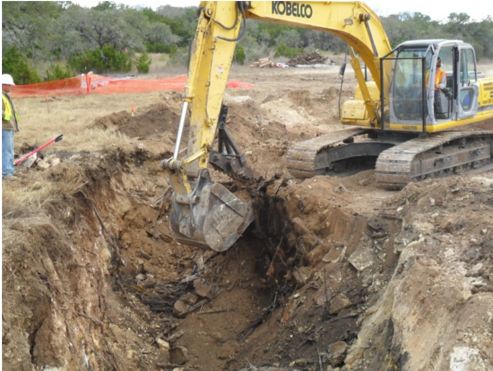
5. Excavation of Trench Ca. View to south, January 2011.
