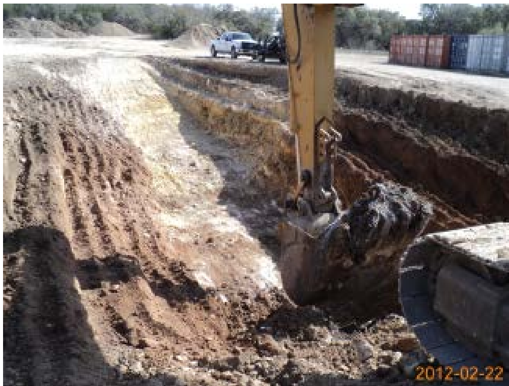
23. Excavation of Trench NT1. View to south, February 2012.
