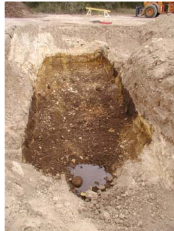
Vegetable Oil applied to Trench 6 (220 gallon tote tanks)
