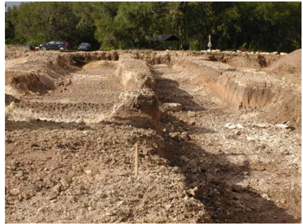
Trench 3 and 4 looking south
