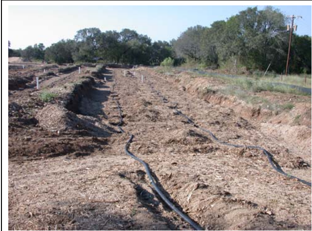
Trench 1 and Trench 2 looking south (irrigation lines within the trenches)
