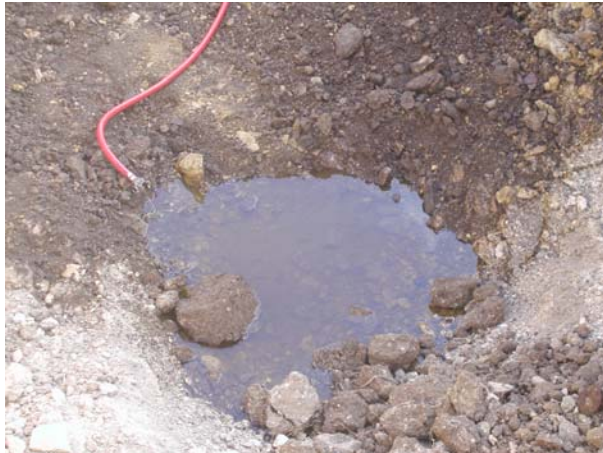
Vegetable Oil applied to Trench 6
