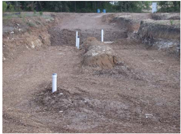
Trench 1 and Trench 2 looking north (4 sumps installed)
