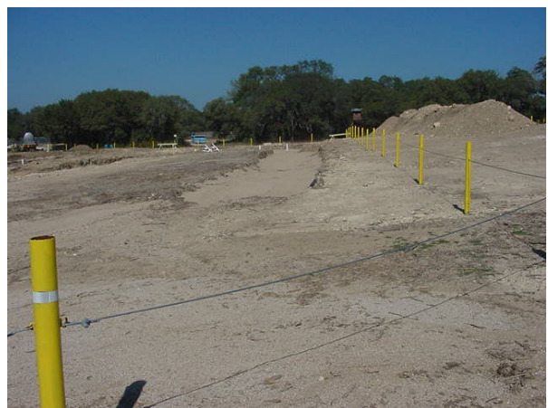
Site security (cable fencing)
