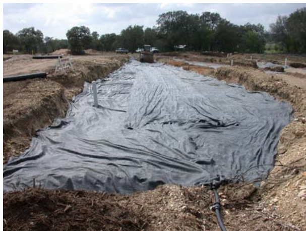
Geofabric layer in Trench 5
