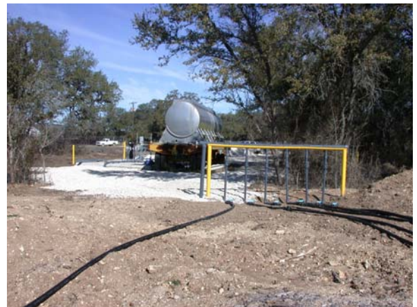
Irrigation tank and distribution system
