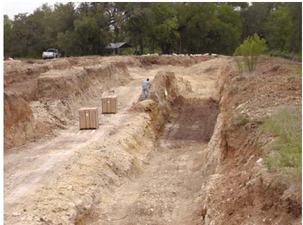
Vegetable Oil applied to Trench 1 (220 gallon tote tanks in trench 2)
