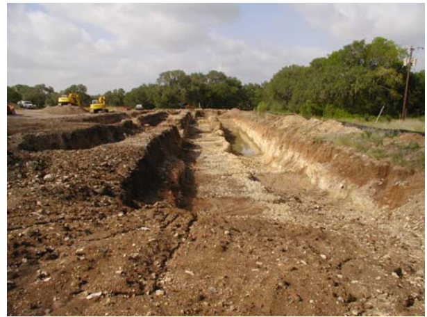
Trenches 1, 2 and 3 looking south
