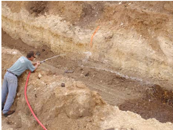
Vegetable Oil applied to Trench 1
