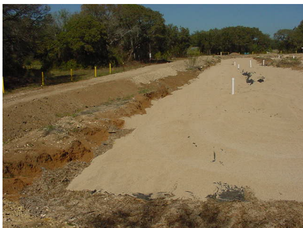
Trench 1 & 2 looking north (berm construction on west side)
