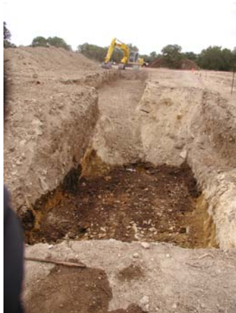
Trench 6 excavation looking south
