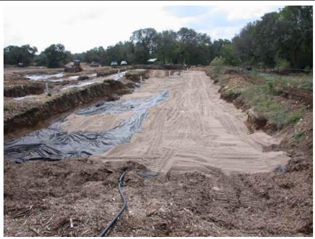
Trench 1 and Trench 2 looking south (geofabric and gravel layer)
