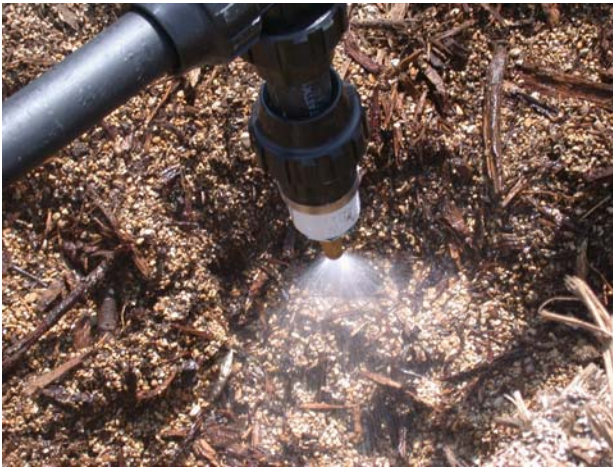
Irrigation spray nozzle testing prior to being covered.
