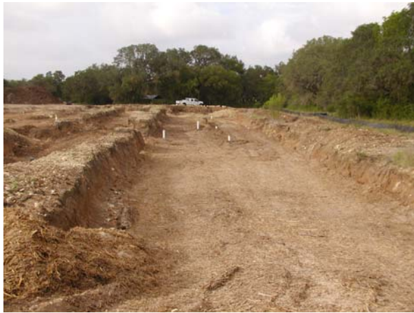
Trench 1 and Trench 2 looking south
