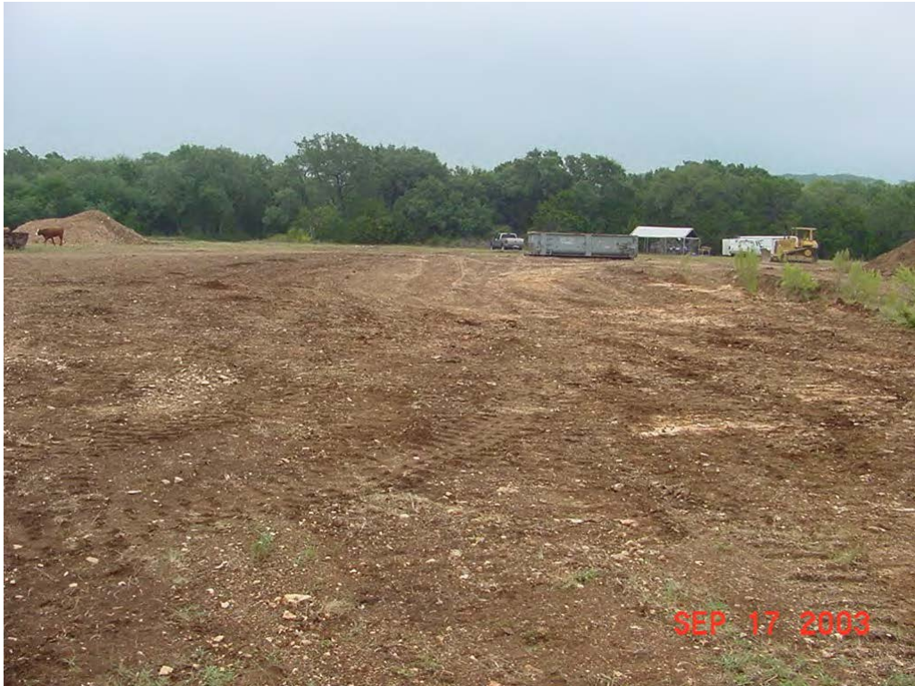
Photo 13-5. Most northern area completely backfilled following September 2003 excavation.
