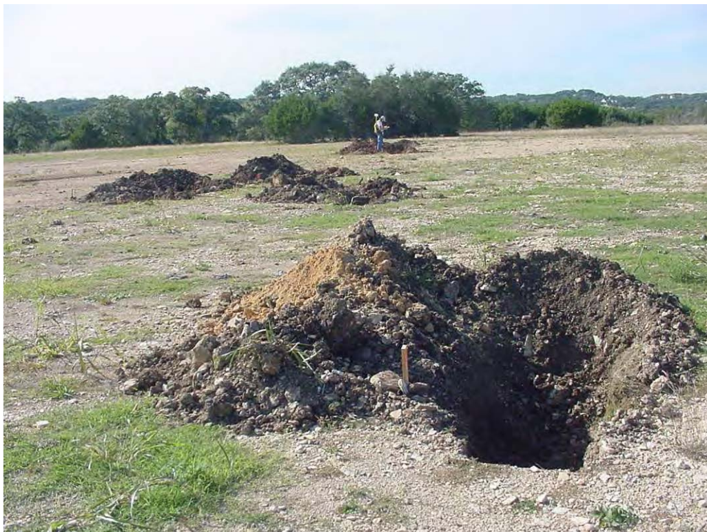
Photo 13-6. Excavation and confirmation sampling in November 2004.
