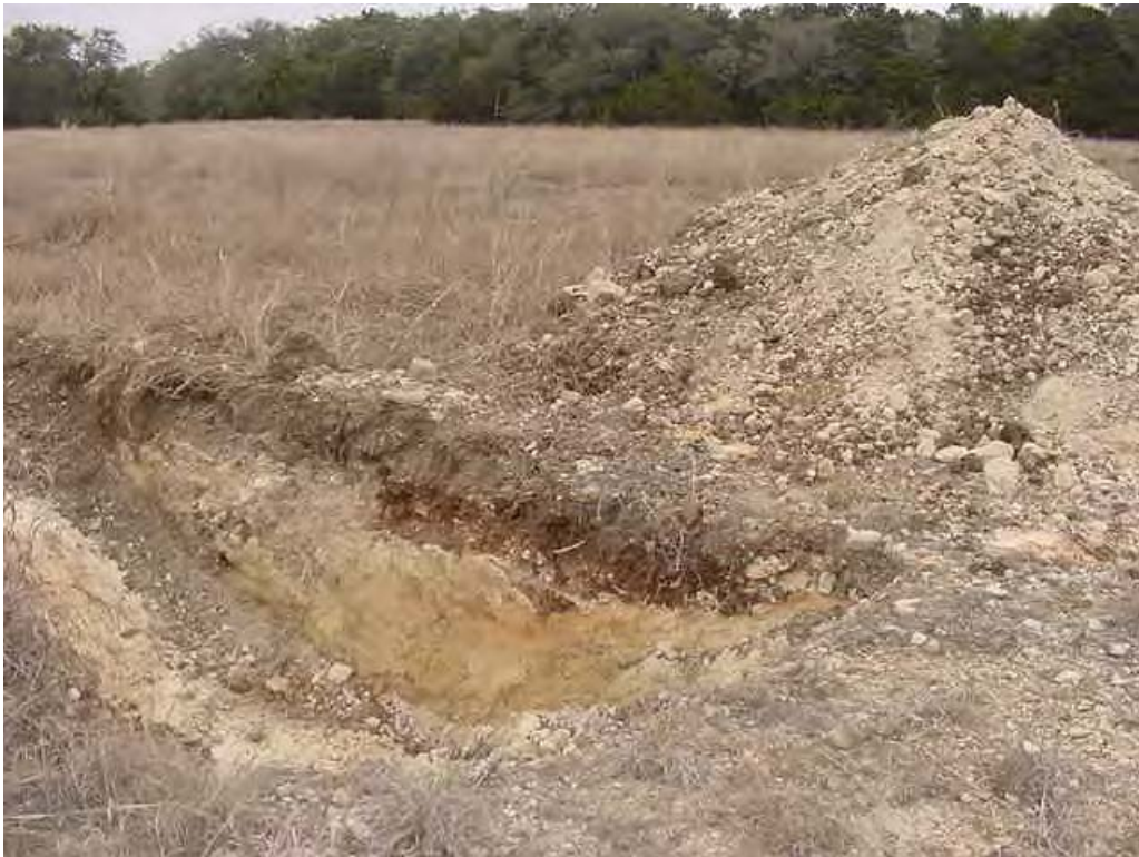
Photo 13-8. Excavation and confirmation sampling of B2-SW14 in March 2008.
