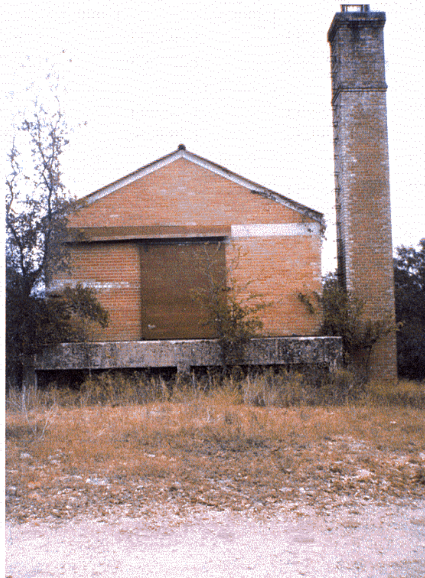
Photo 6: I-1, inactive incinerator building.
