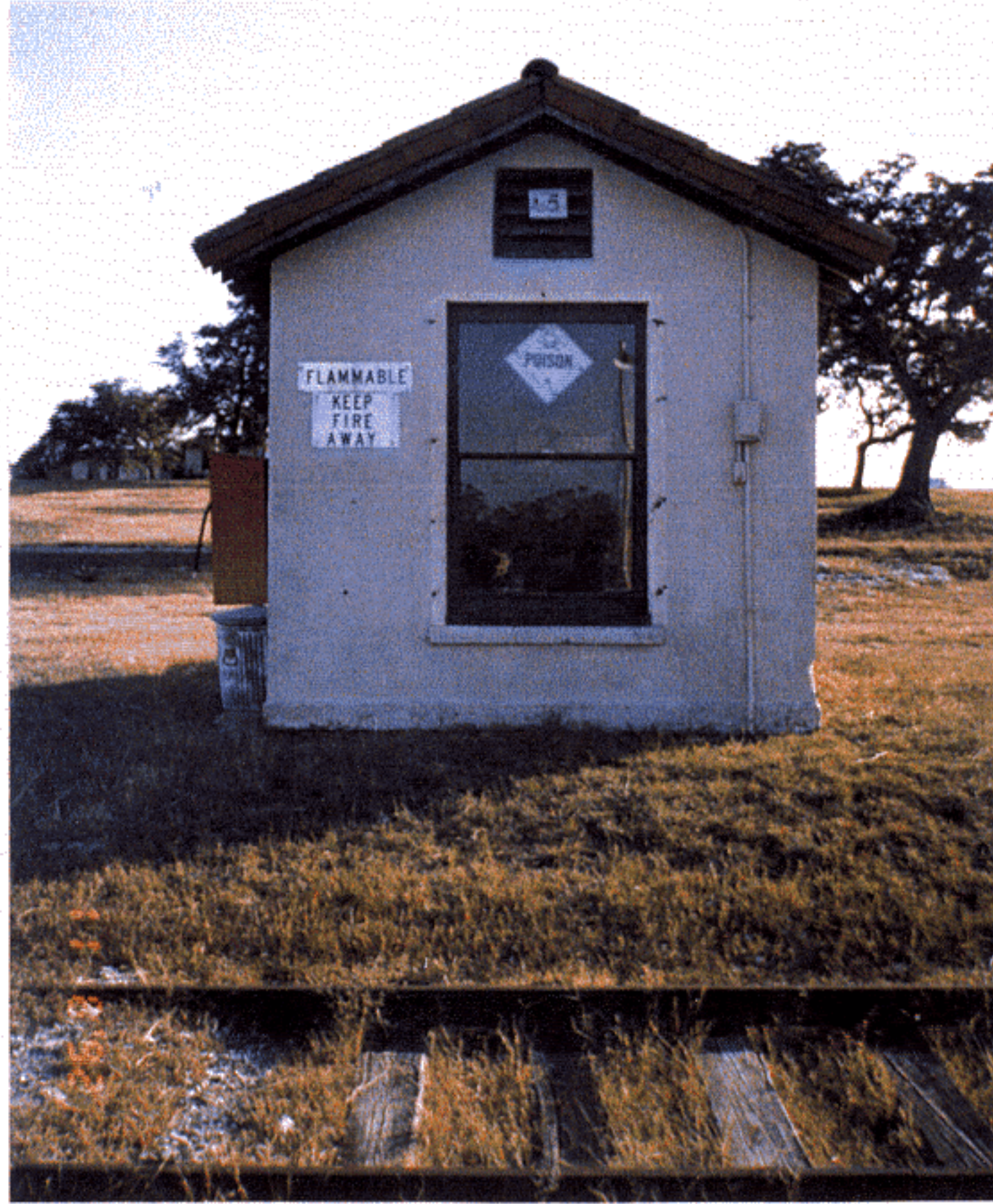
Photo 5: Current pesticide storage building.
