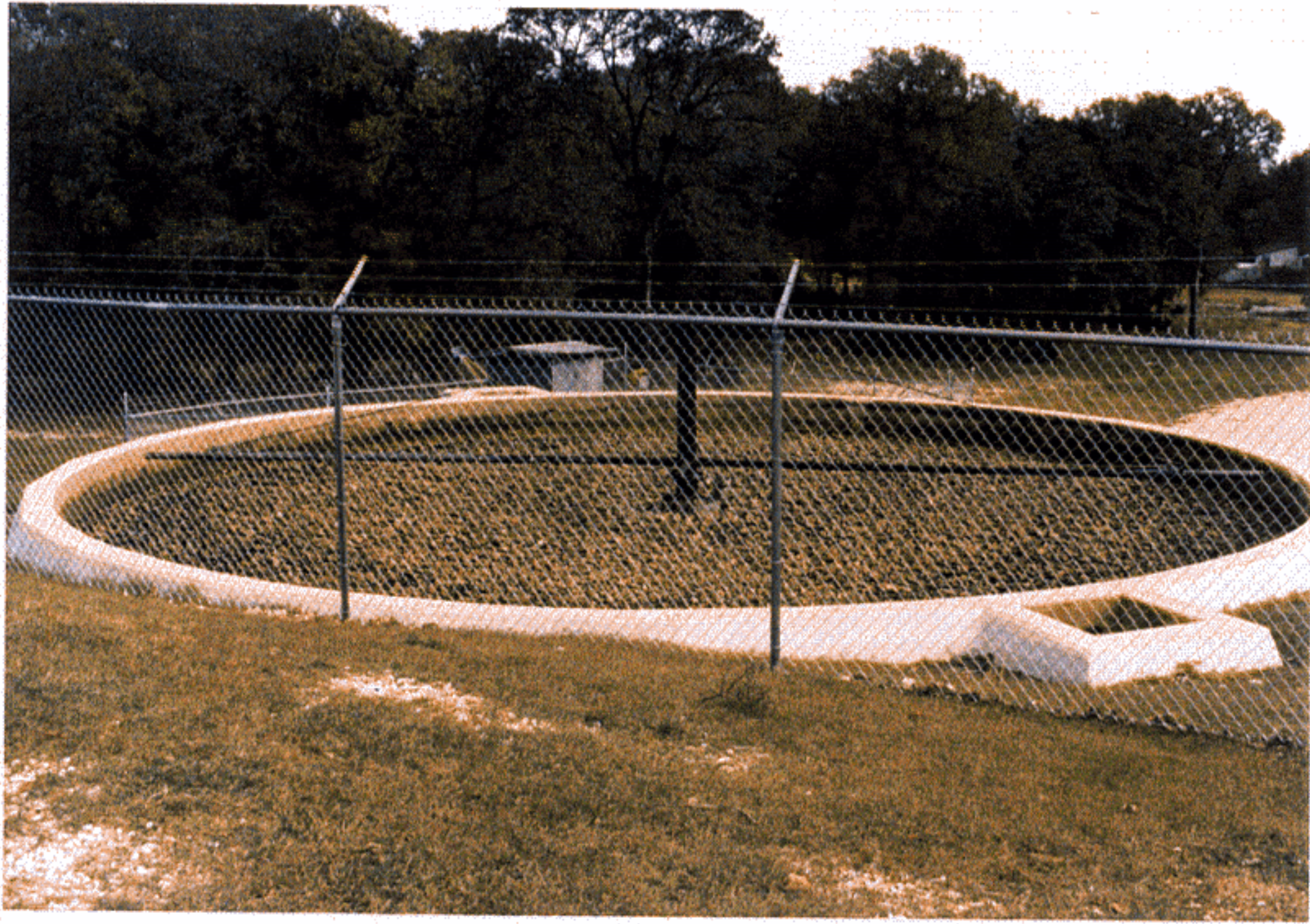
Photo 31: Trickling filter at wastewater treatment plant.
