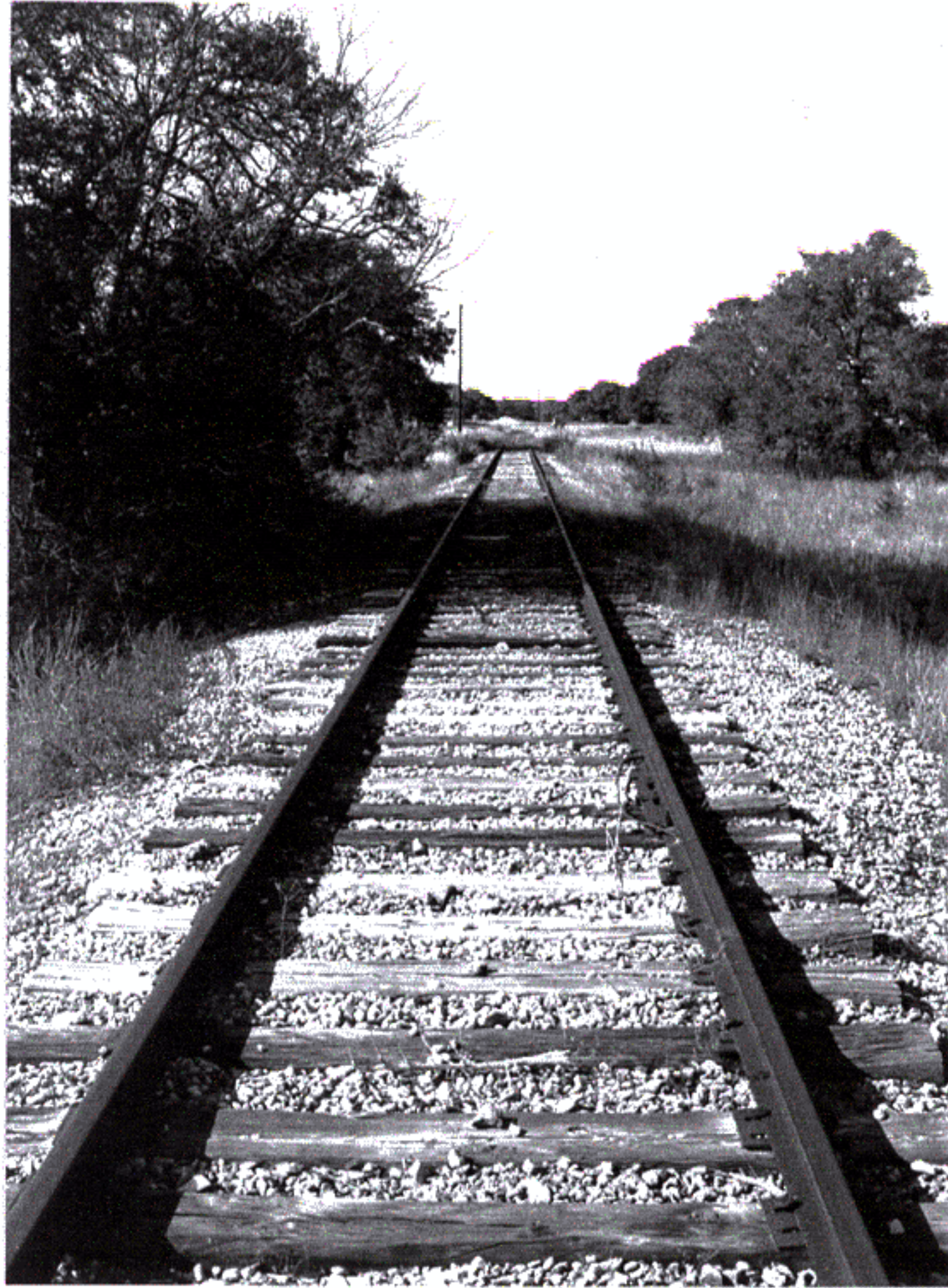
Photo 1: Railroad track through CSSA.
