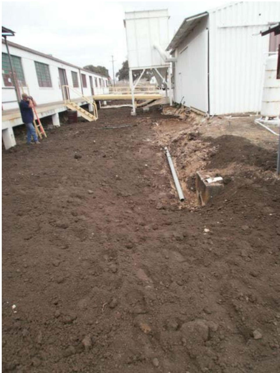
Photo 8. AOC-65 Top Soil Replacement near Building 90. (Photo taken 01-11.)
