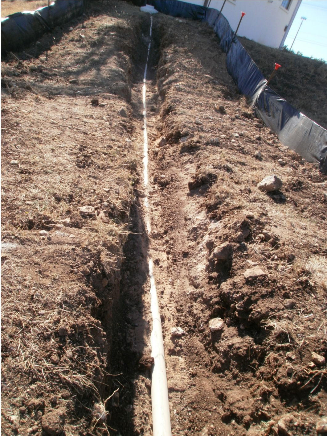
Photo 1. Bldg. 89 Sanitary Sewer Line Exposed. (Photo taken 12-10.)
