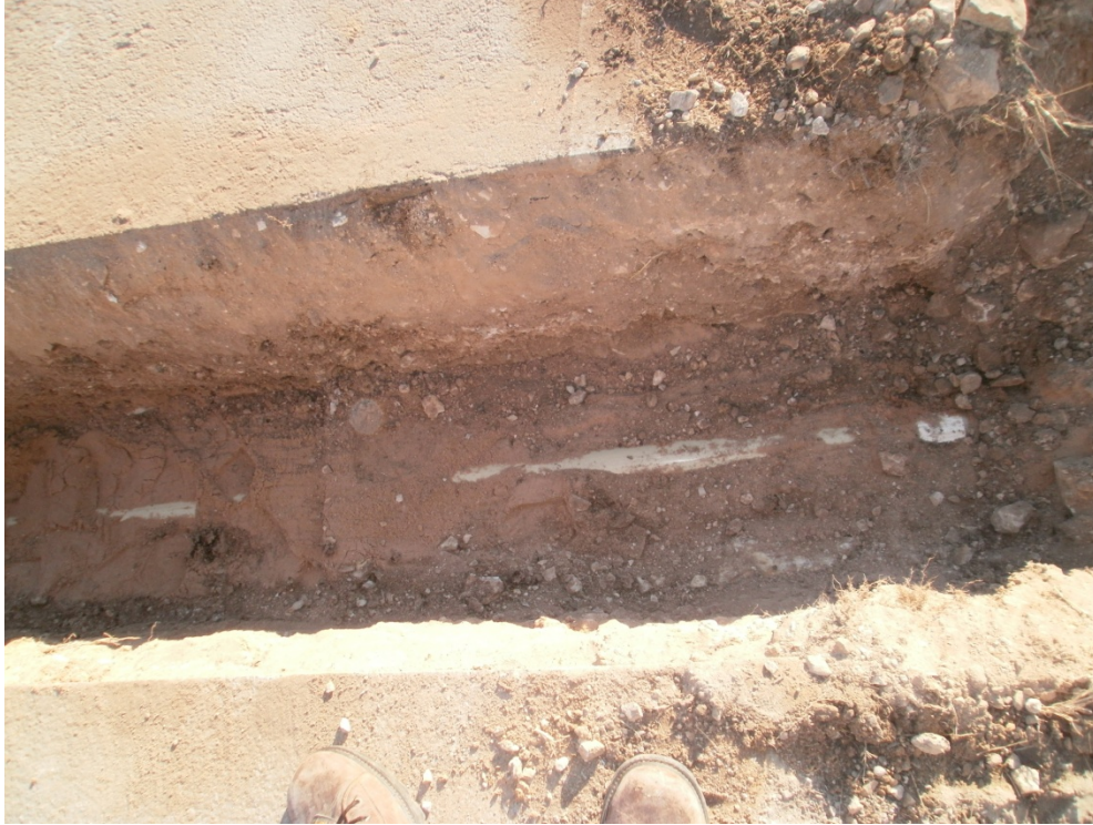
Photo 2. Building 90 sand bedding materia (Photo taken 12-10.)
