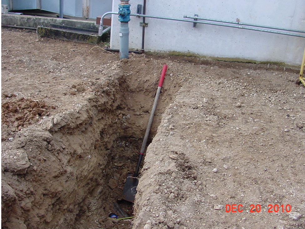
Photo 5. Sanitary Sewer Line Location near Building 90 Test Fire Room. (Photo taken 12-20-10.)
