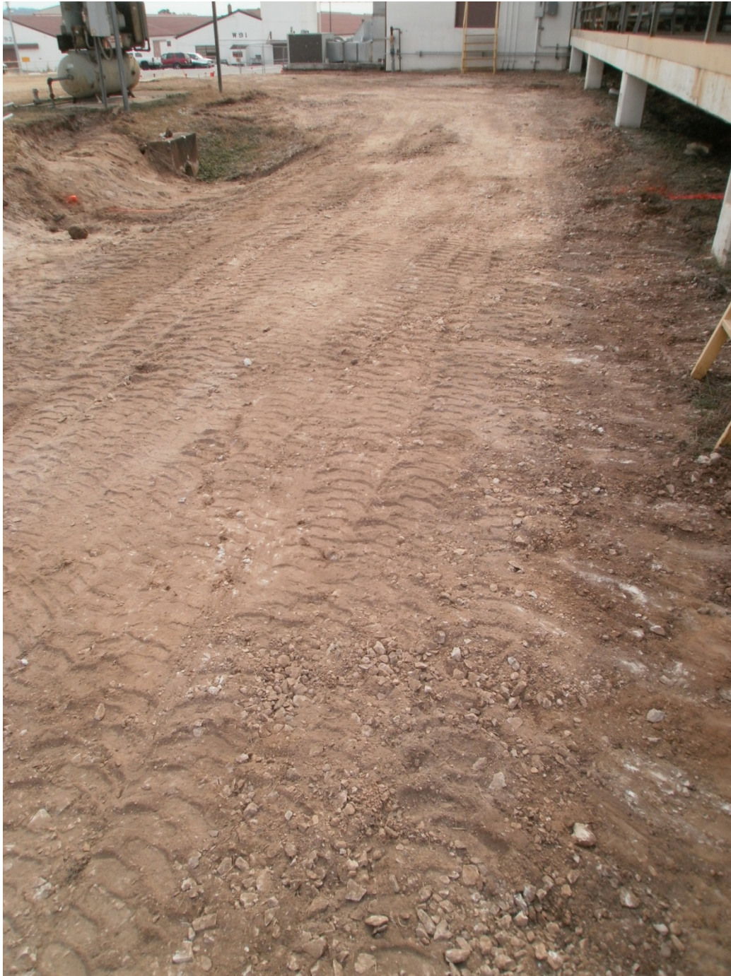
Photo 7. AOC-65 Surface Soil removal near Building 90. (Photo taken 12-10.)
