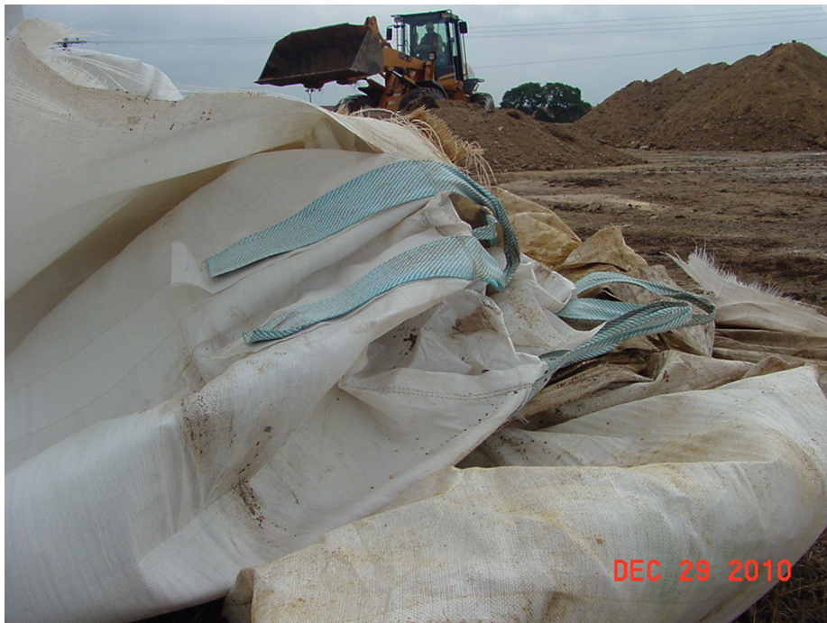
Photo 6. PIMS mixing near Building 89. (Photo taken 12-29-10.)
