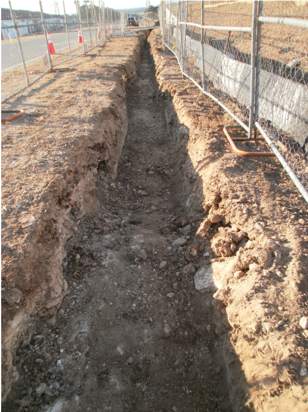
Photo 4. Sand Bedding material Removed near Building 90 (Photo taken 12-10.)
