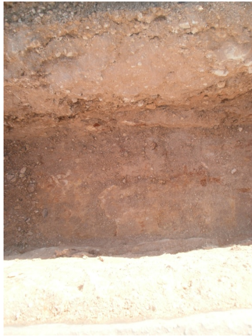
Photo 3. Removed sand bedding material (Photo taken 12-10.)
