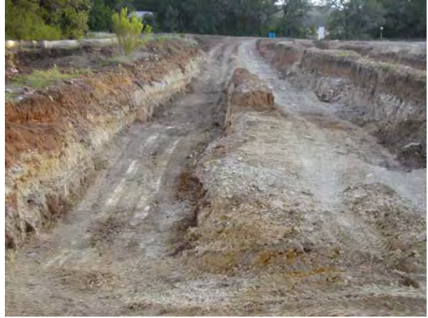
Trench 1 and Trench 2 looking north
