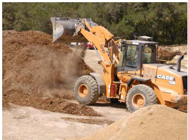
1/4" Gravel and Tree mulch mixing
