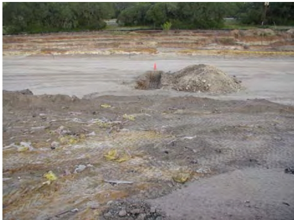
Trench 6 investigation (PIMS mixing in soils from trench 5 in foreground)
