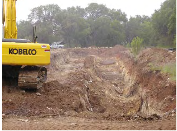
B-3 Trench 2 (left), Trench 1 (right)
