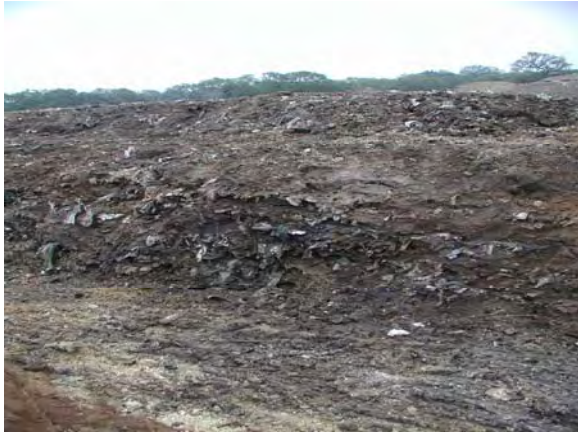
B-3 Landfill Sidewall of Trench 1
