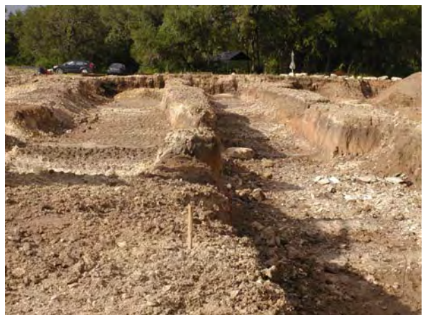
B3 Trenches 3 and 4
