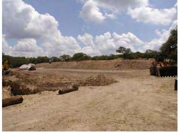
B-3 Trench 4 stockpiles (Trench 3 stockpiles #10 & #11 covered in plastic)
