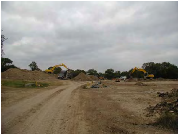
B-3 Trench 1 material loaded into trucks
