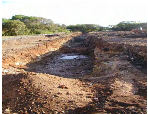
B-3 Trench 1 looking north
