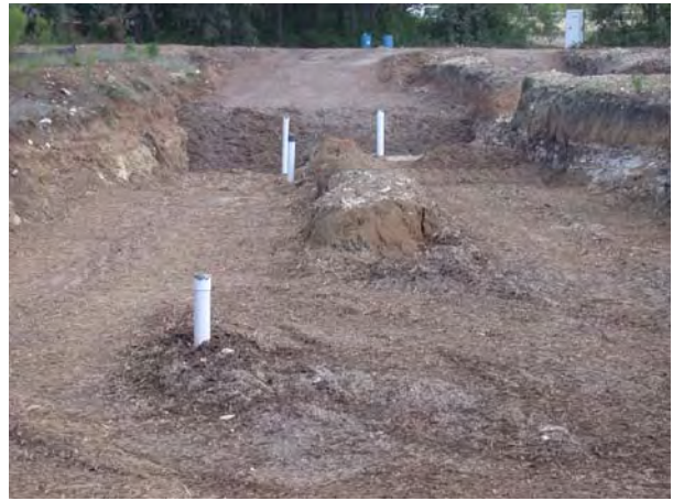
Trench 1 and Trench 2 looking north (4 sumps installed)
