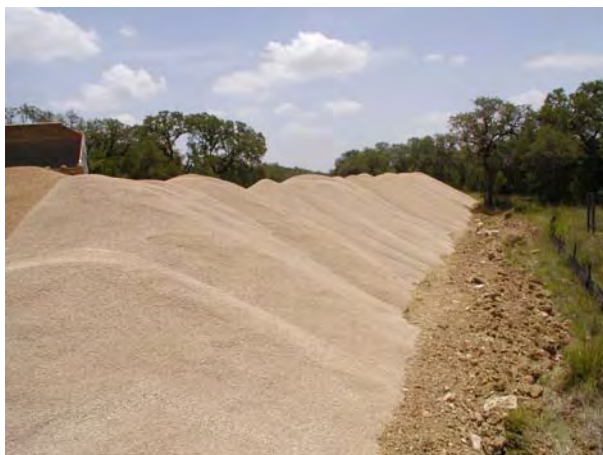
Gravel for Bioreactor
