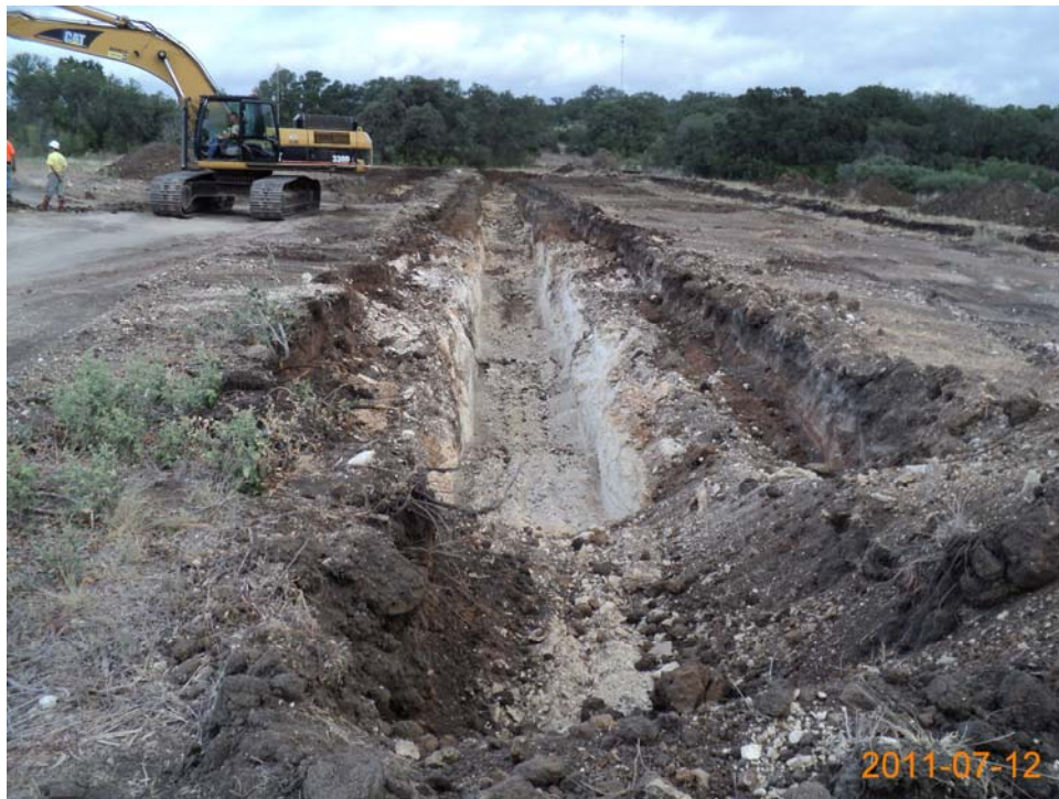
Photo 5. Excavated Trench 2, looking northwest (July 2011).
