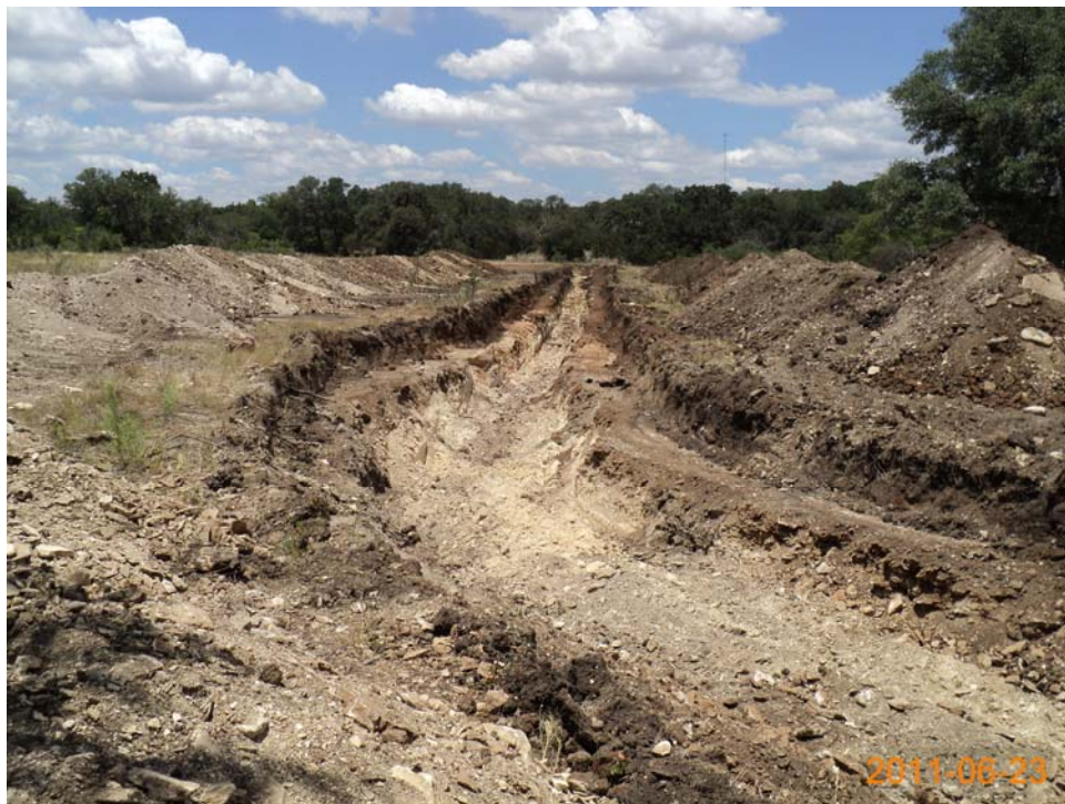
Photo 4. Excavated Trench 1, looking northwest (June 2011).
