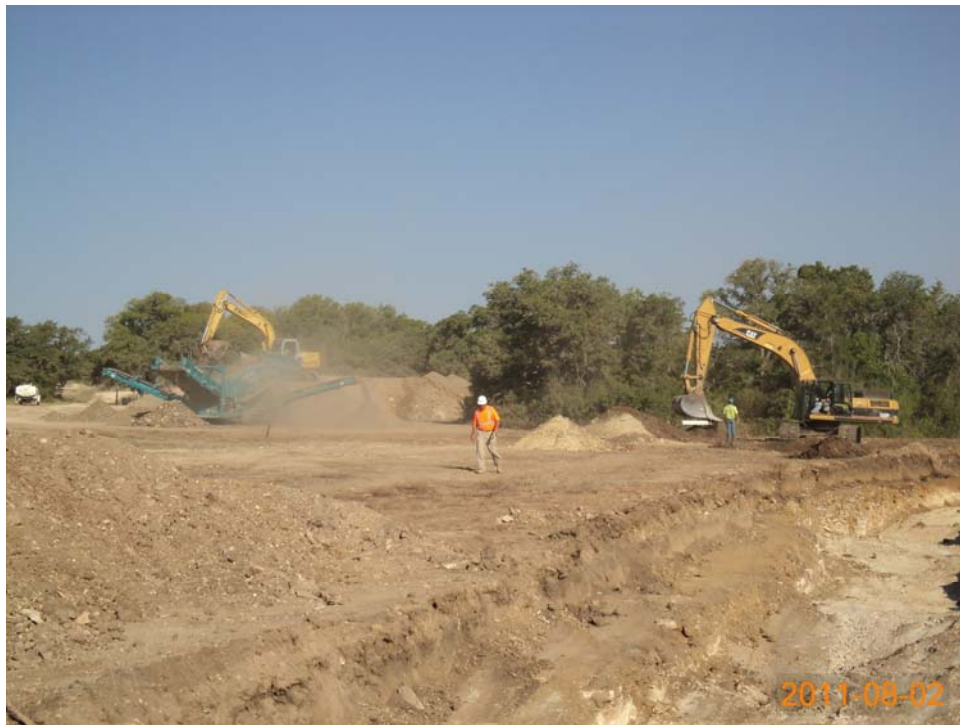
Photo 3. Excavation at SWMU B-27, looking west (August 2011).
