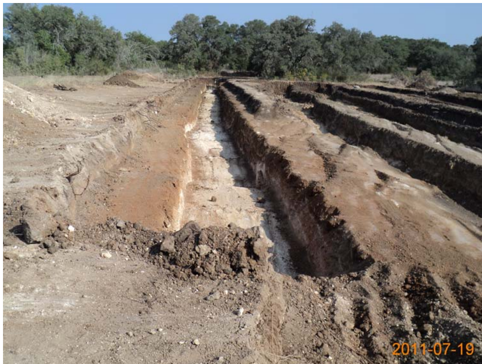
Photo 6. Excavated Trench 5, looking northwest (July 2011).
