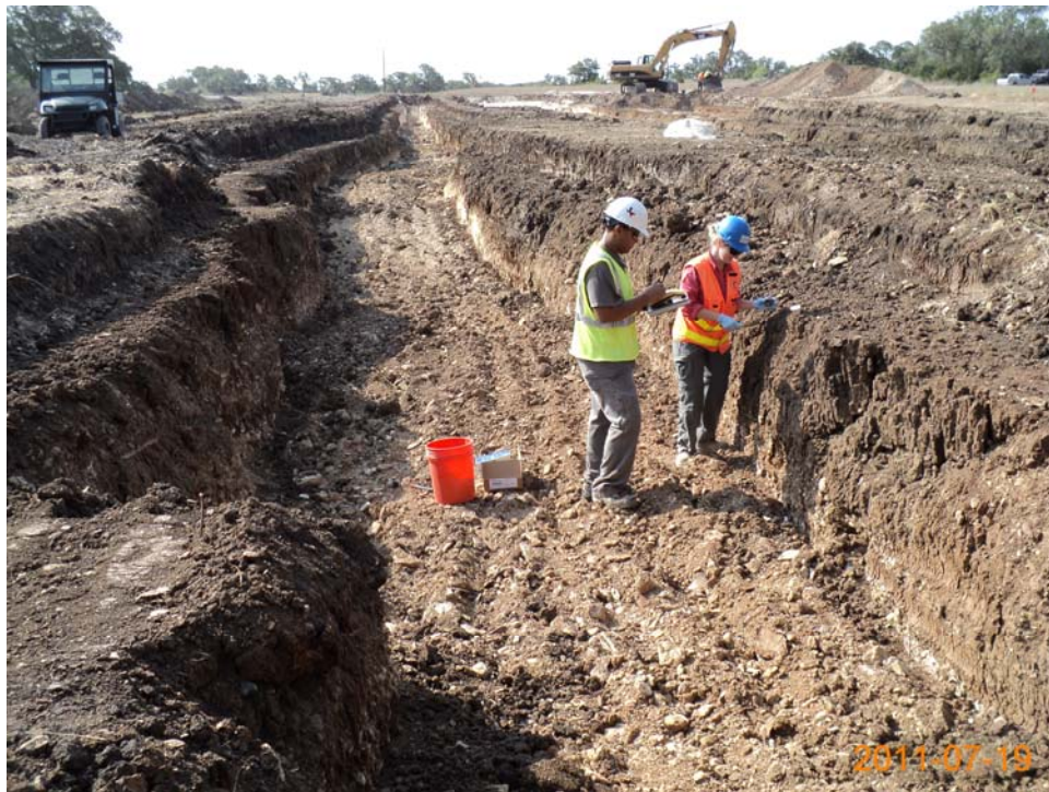
Photo 9. Confirmation sampling at Trench 1, looking southeast (July 2011).
