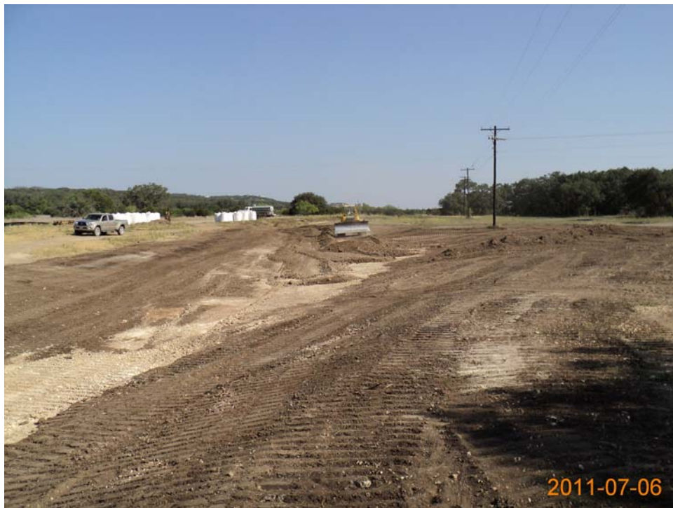
Photo 10. Final graded site, looking west (July 2011).
