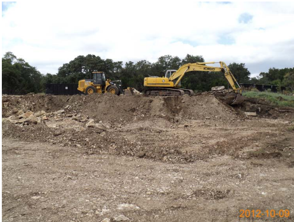
Photo 3. SWMU B-13 south end excavation, looking east (October 2012).
