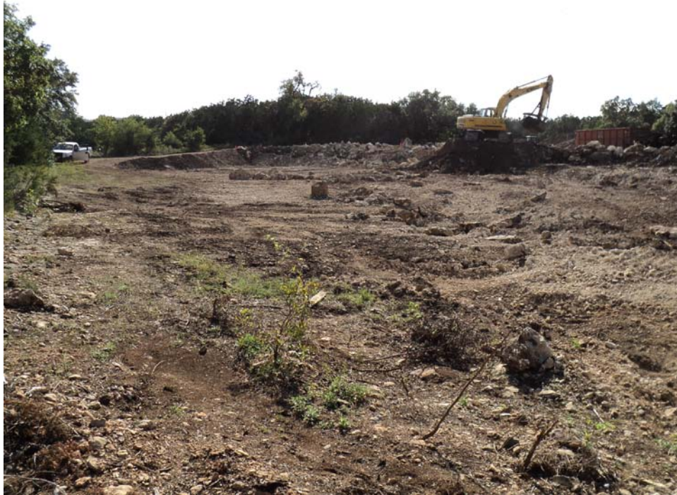
Photo 1. SWMU B-13 north end excavation, looking north (October 2012).
