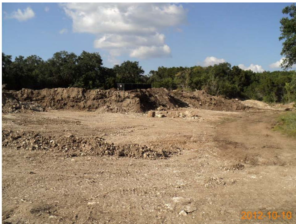
Photo 4. Completed excavation, north end of site, looking north (October 2012).
