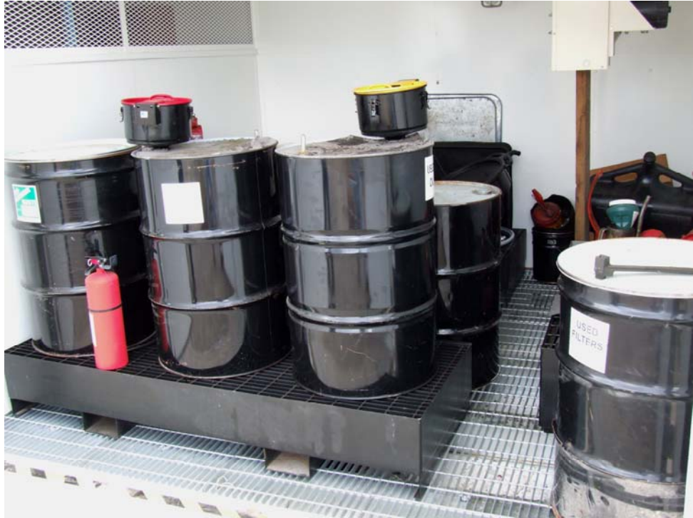
Figure 2 - Interior of used oil and gasoline storage container outside Bldg 4 Motor Pool.
