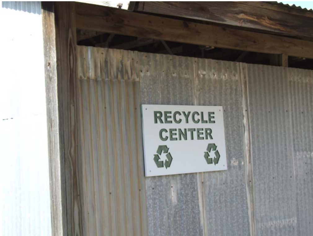
Figure 1 - Recycling Collection Center at Bldg 302
