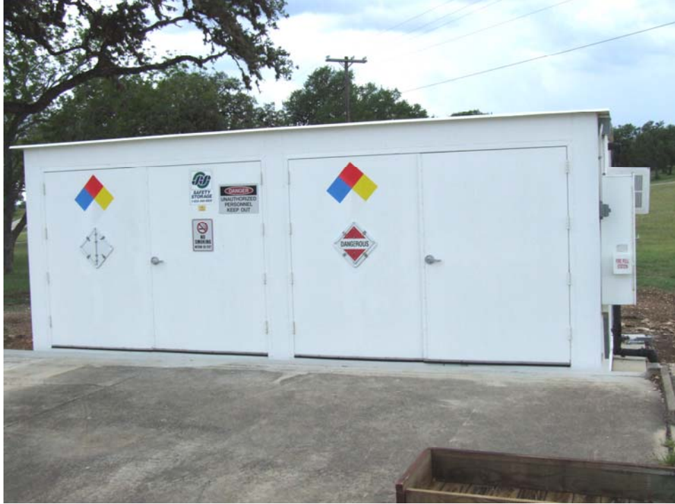
Figure 1 – Exterior of used oil and gasoline storage container outside Bldg 4 Motor Pool.
