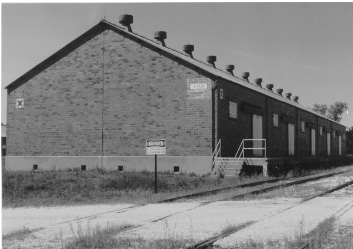
Figure 27. Hollow clay tile aboveground magazine.
