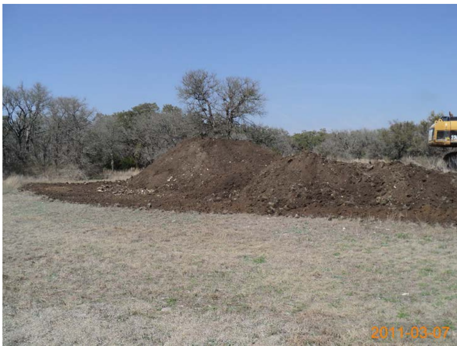
Photo 12. Excavation of AOC-59, looking west. (March 2011)
