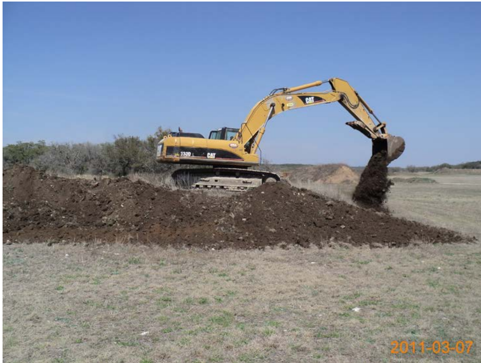
Photo 13. Excavation of AOC-59, looking north. (March 2011)
