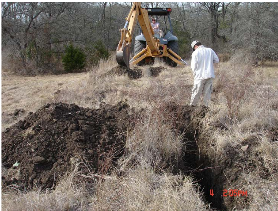
Photo 5. AOC-59 (test trenching in the soil mound area). (January 2006)
