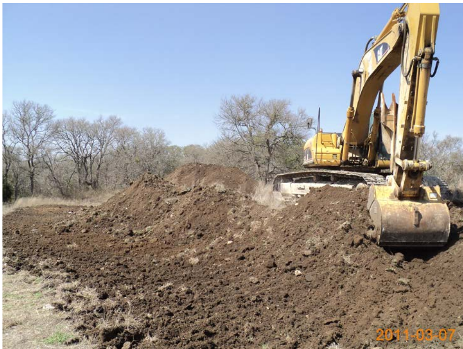
Photo 14. Excavation of AOC-59, looking west (March 2011)
