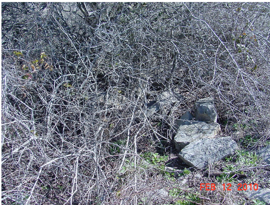
Photo 11. AOC-59 partially buried old stone wall. (February 2010)
