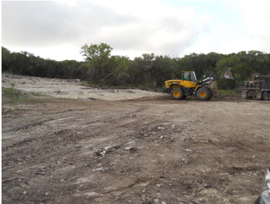
Photo 5. AOC-51 after excavation, looking southeast (May 2012).
