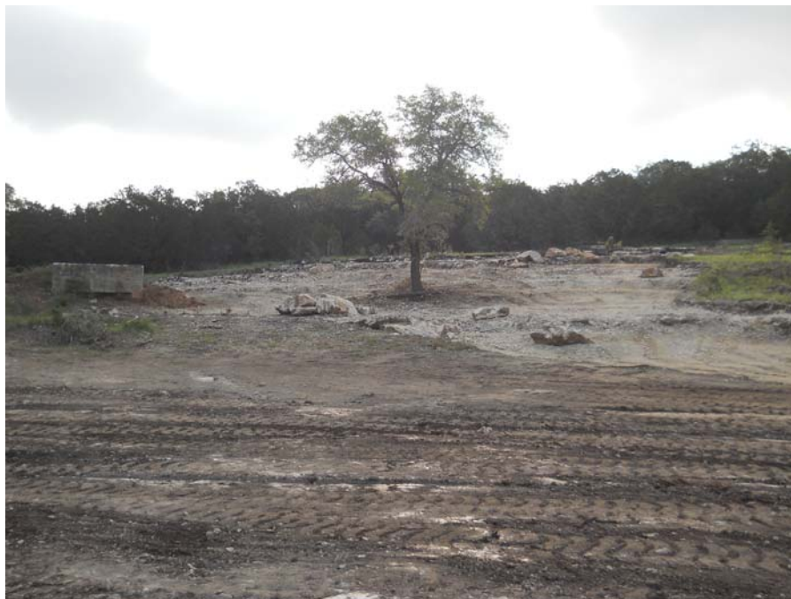
Photo 4. AOC-51 after excavation, looking northeast (May 2012).
