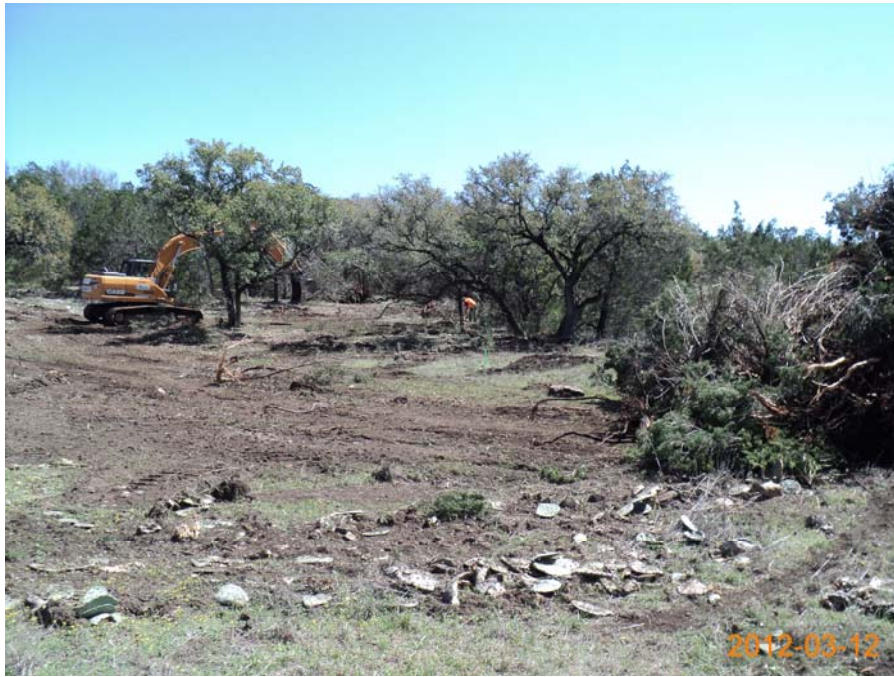
Photo 3. Excavation of AOC-51, looking northwest (March 2012).
