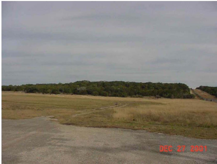
Photo 1. View of AOC-51, looking northeast (December 2001).
