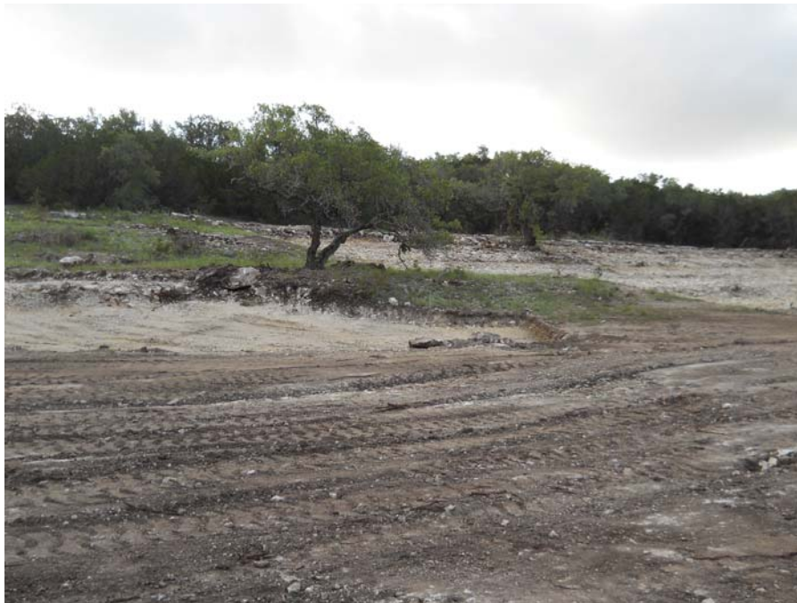
Photo 6. AOC-51 after excavation, looking southeast (May 2012).
