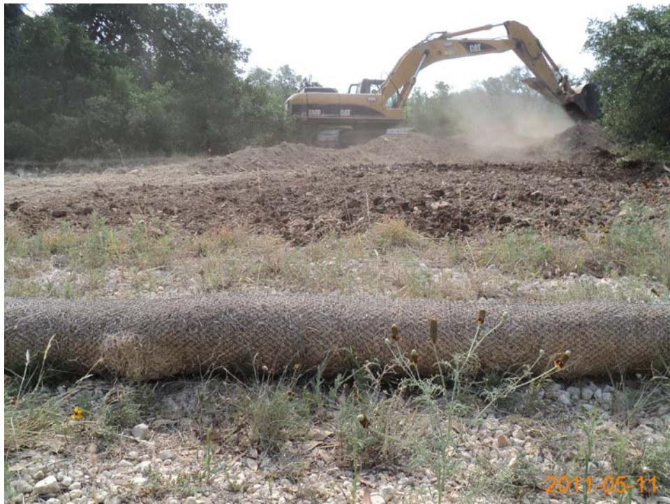
Photo 5. Excavation of AOC-45, looking south (May 2011).
