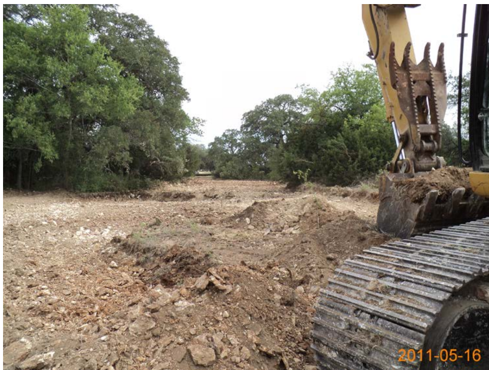
Photo 6. Excavation of AOC-45, looking north (May 2011).
