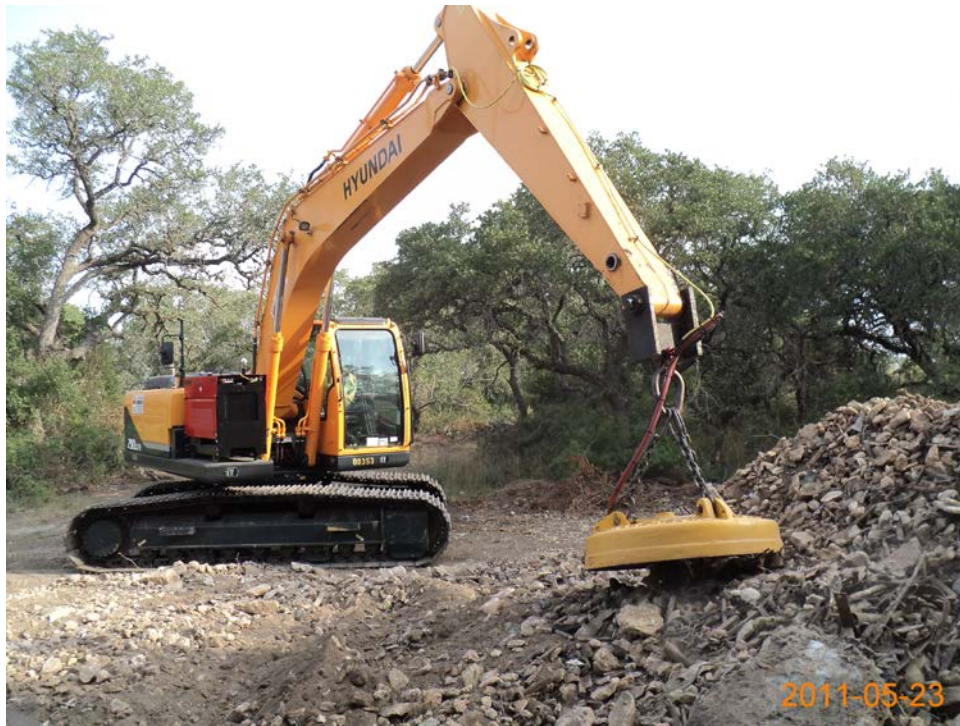
Photo 5. Excavator with magnetic attachment sorting debris at AOC-42 (May 2011).
