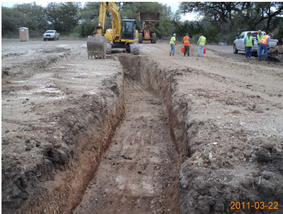
Photo 10. Excavation of Trench 4 at AOC-62, looking east (March 2011).
