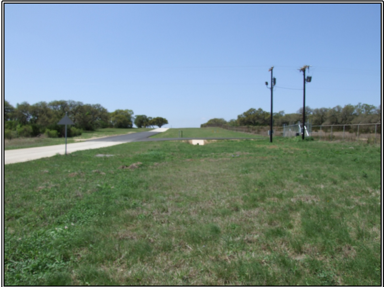
Figure 2B-6: View of North Outer Road easement to the north adjacent to SWMU B-71, looking west.
